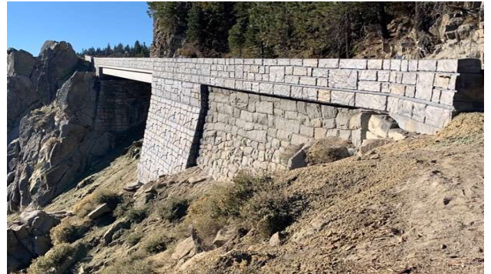
FIGURE 18: Completed Echo Summit Bridge
