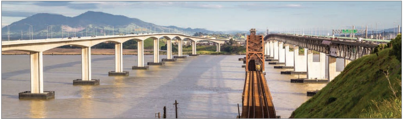
FIGURE 15: New Benicia-Martinez Bridge Is Designed to Meet Highest Standards
