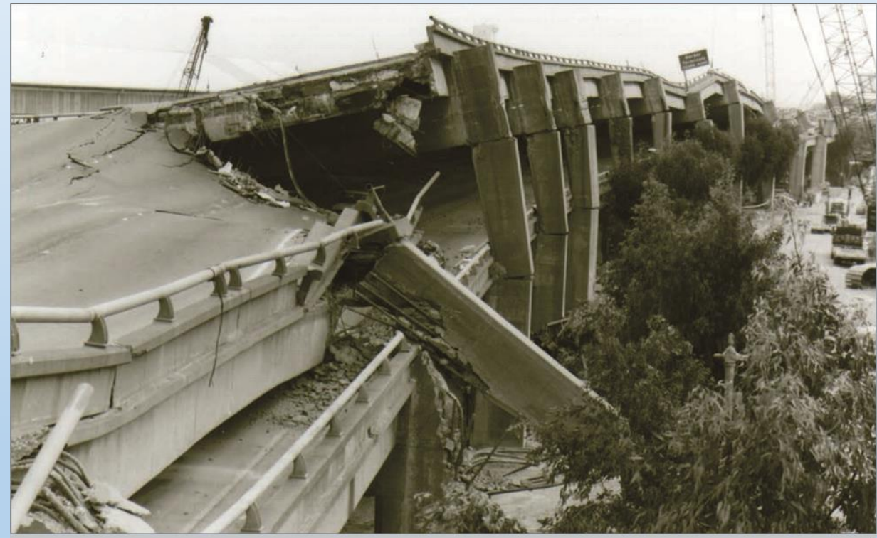
FIGURE 7: Collapsed Section of the Cypress Street Viaduct
