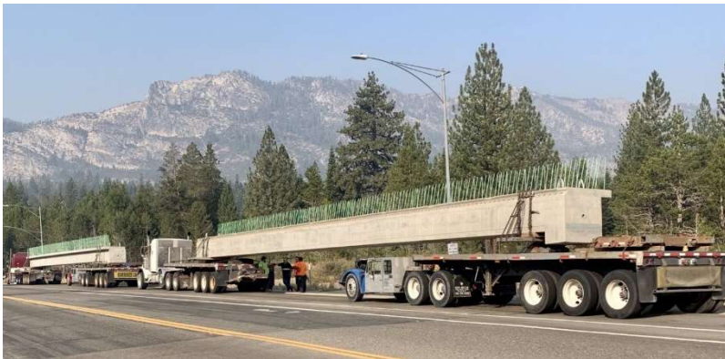
FIGURE 17: Echo Summit Precast Girders
