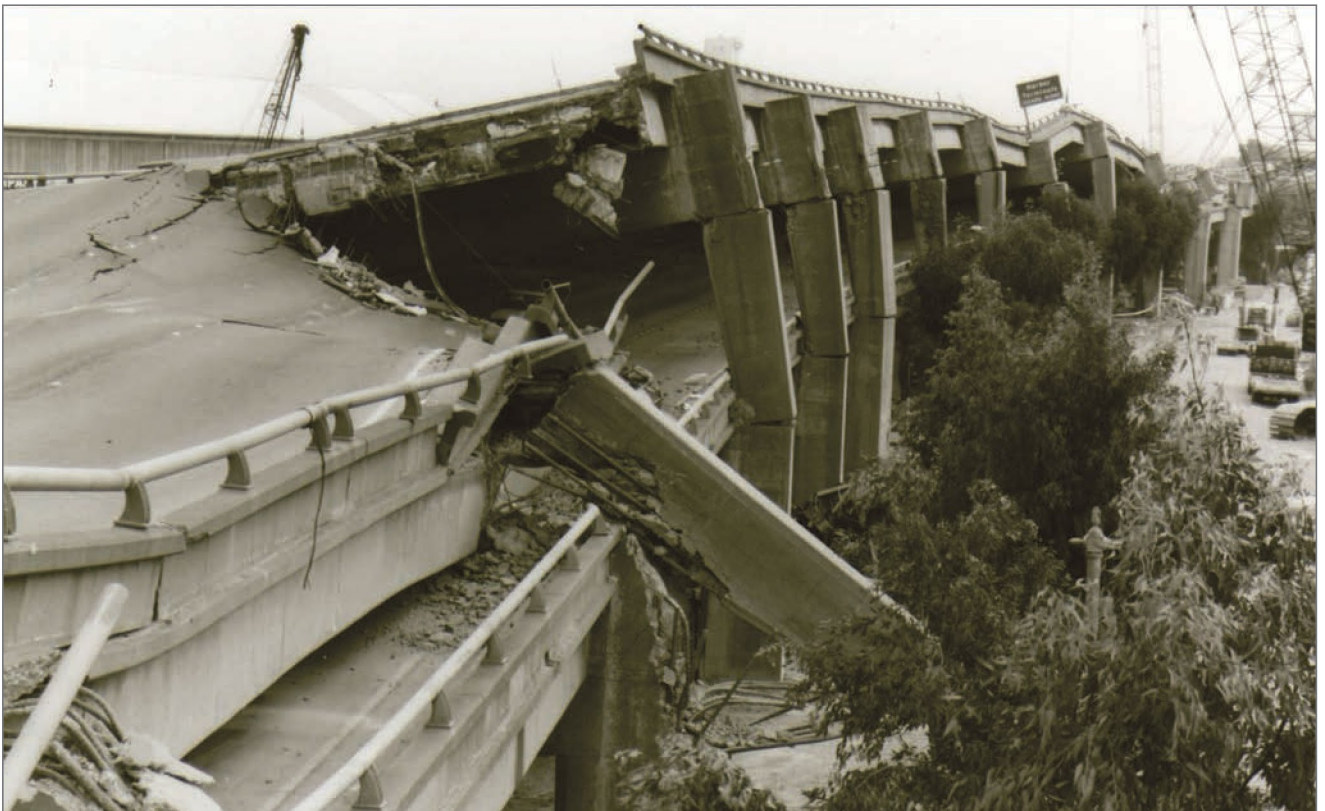
FIGURE 7: Collapsed Section of the Cypress Street Viaduct
