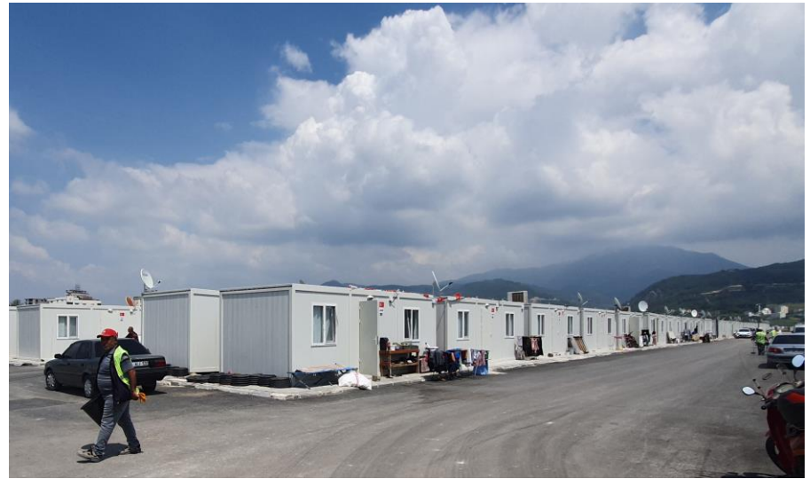
Container city in Osmaniye province
