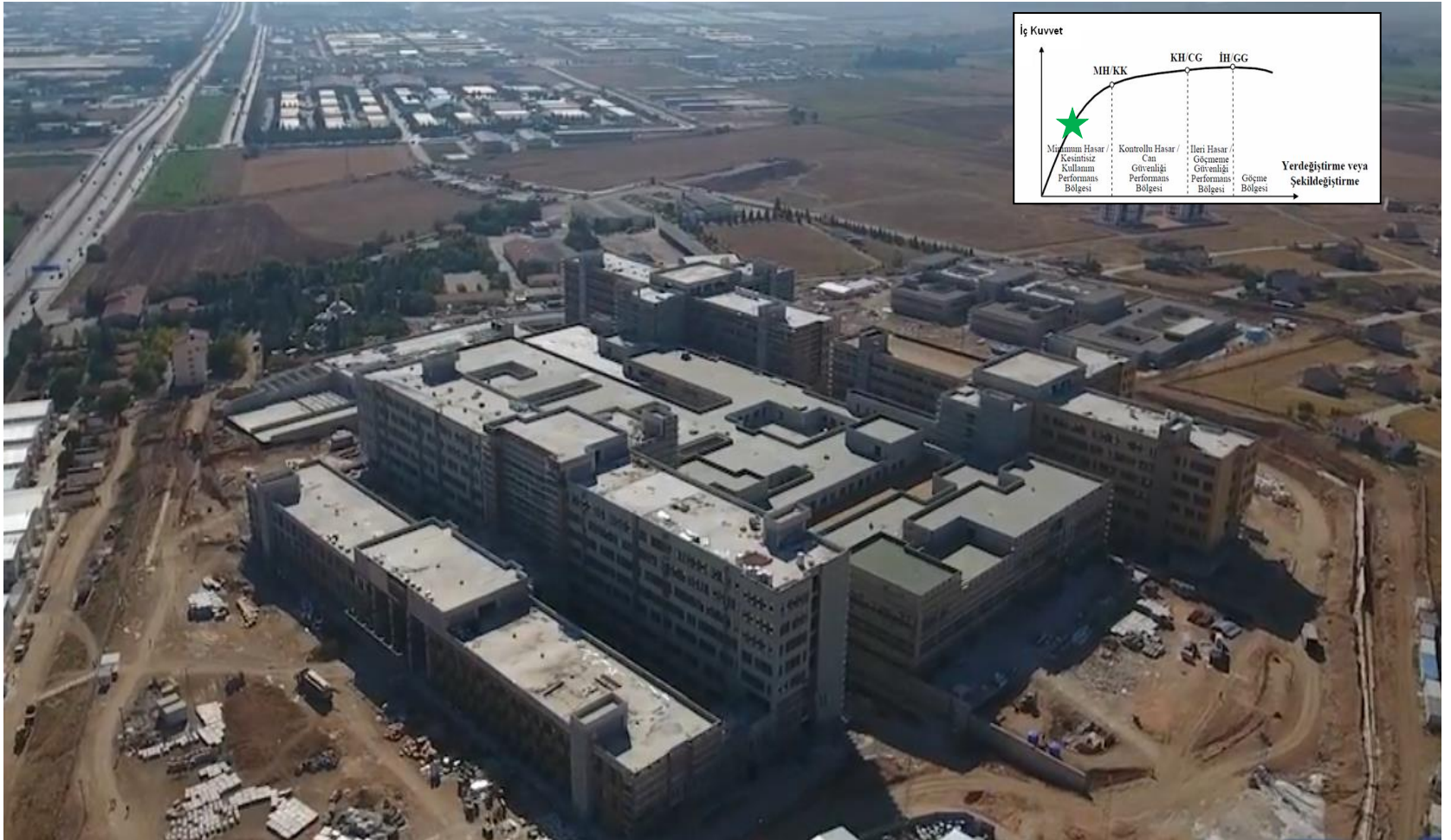
Eskişehir City Hospital | 2017 | 330,000 m 2 | 1081 Bed | 973 FPS Isolator
