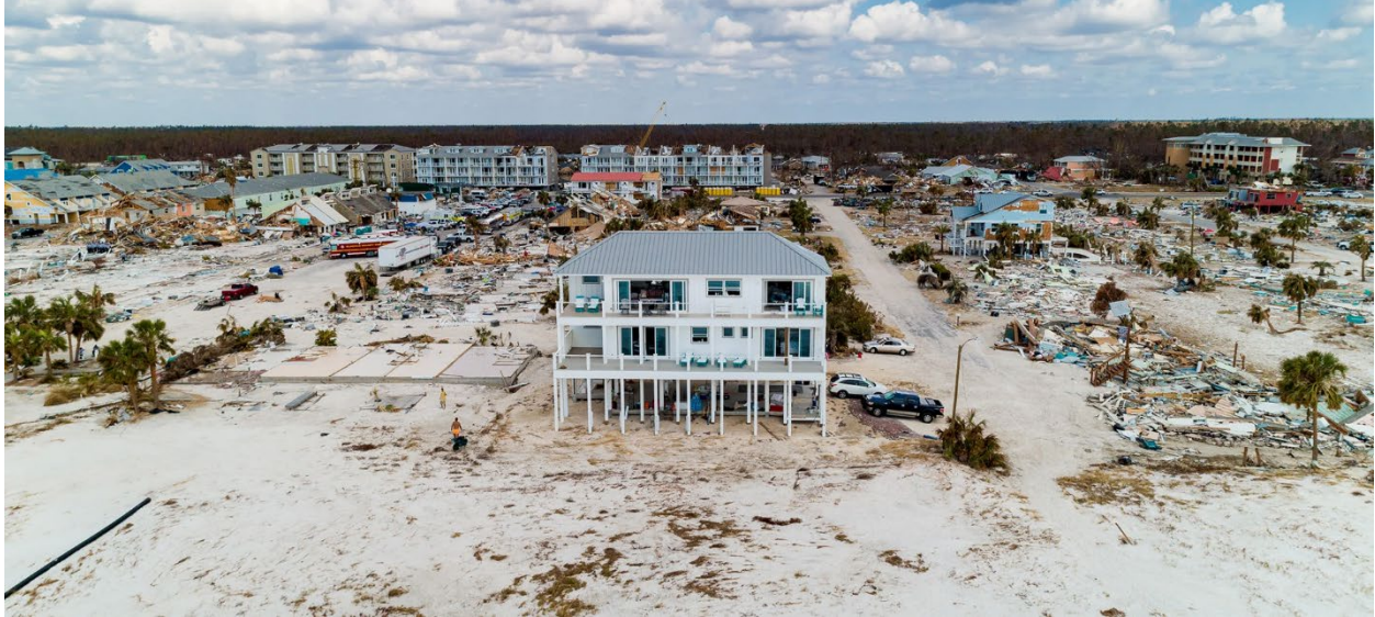
Figure 3.23 – Building survived 2018 Hurricane Michael winds and storm surge in the Florida panhandle, due to being properly mitigated for flood and lateral wind loads.
