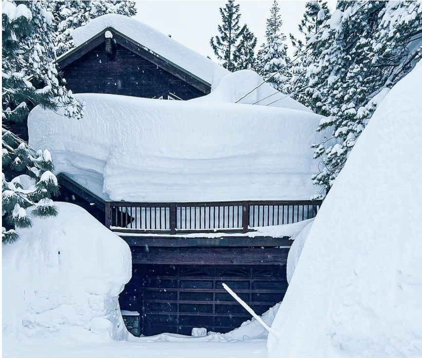
Figure 3.28 – Snow load causing beam over garage door to sag. South Tahoe Snow Load Damage. Photo courtesy Brandon Miller.
