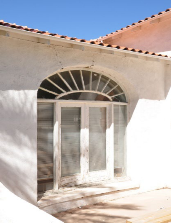
Figure 4.27 – Cracks in archway of adobe house. Photo courtesy Fred Turner, EERI.
