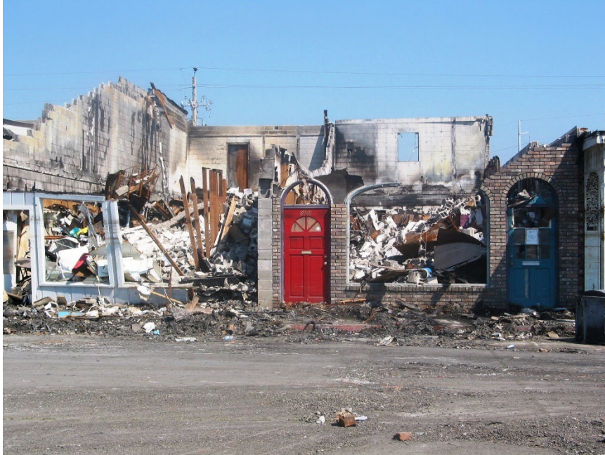
Figure 3.21 – Hurricane Katrina tore the roof off this building, and began destroying the building's three unreinforced masonry walls. Storm surge flooding filled the building up to about seven feet high, and part of the building above the water line caught on fire. This photo shows that the door is still intact. Photo courtesy Raymond Lui.
