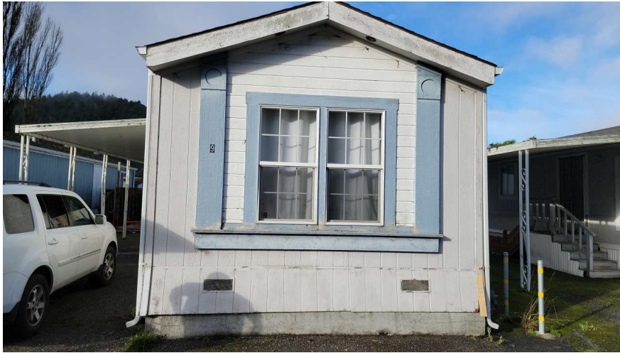
Figure 3.42 – Manufactured home survived 2022 Ferndale Earthquake. Shifted one inch on its foundation. Tagged INSPECTED. Photo courtesy Gurbir Singh.
