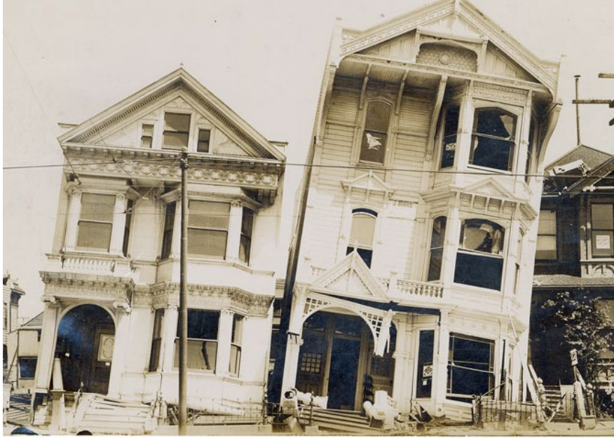
Figure 3.82 – Liquefaction causes tilting of these Victorian homes.
