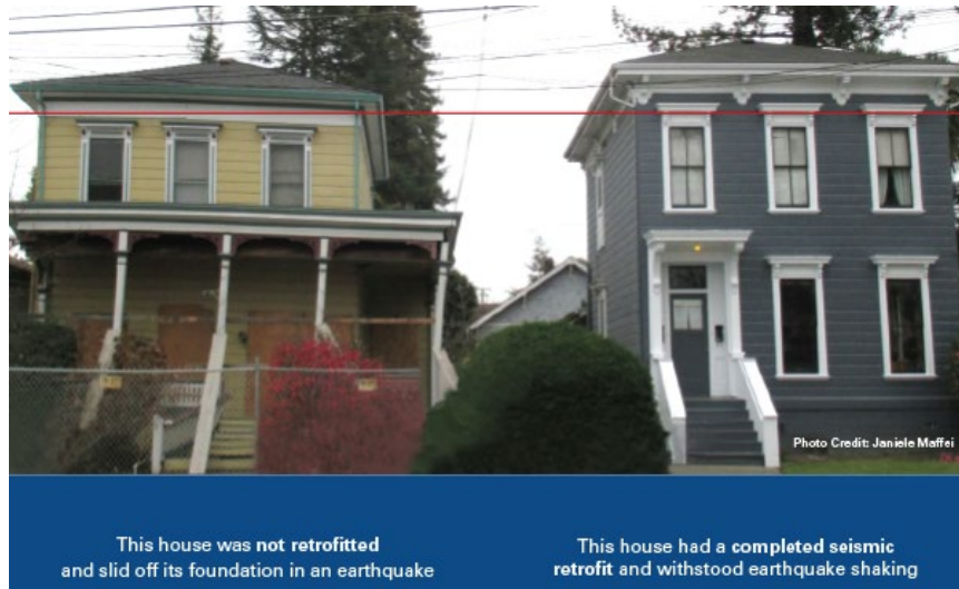
Figure 3.67 – Example of two homes side by side; left house had no seismic retrofit work and suffered damage, while the right house was completely retrofitted and suffered no damage.
