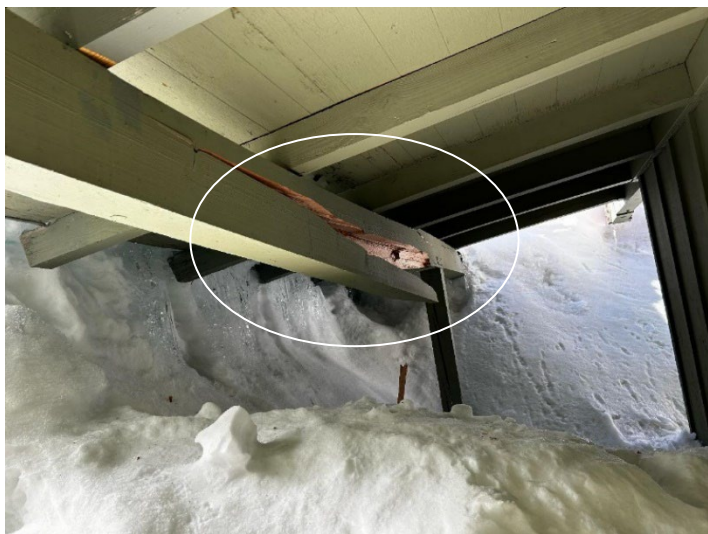
Figure 3.45 – Wood beam across front porch cracked due to snow load. House was tagged RESTRICTED USE to prevent use of front door. 2023 Mono County Snow Load Mission. Photo courtesy Gurbir Singh.
