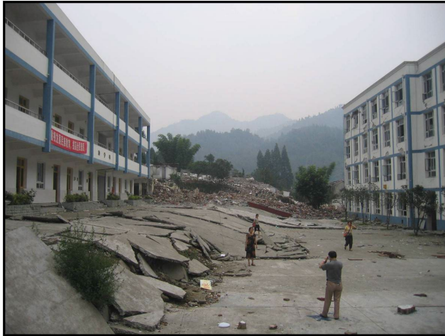
Figure 4.3 – Scarp developed between two apartment buildings in Taiwan, possibly due to faulting.
