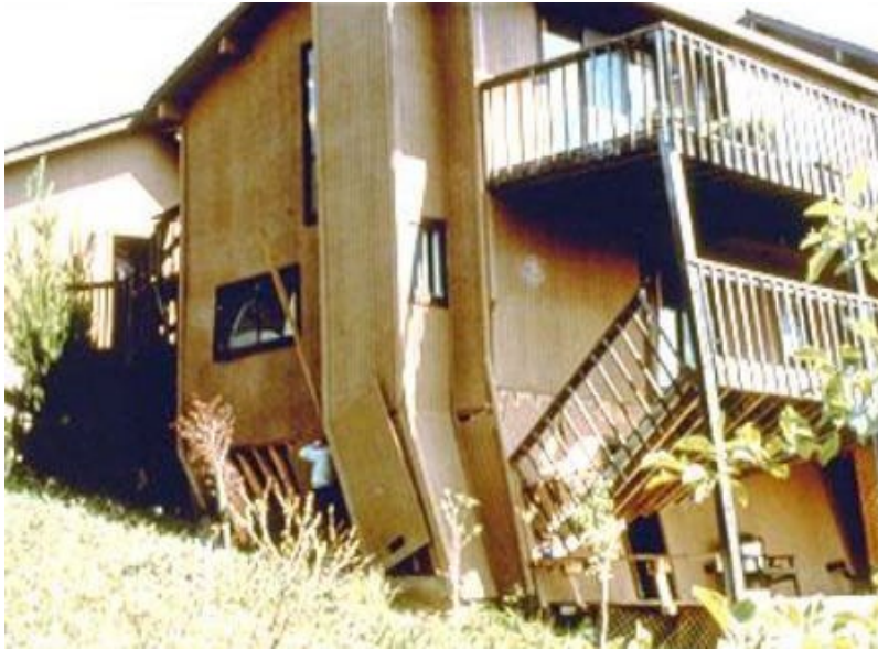
Figure 3.88 – Soft story damage to apartment building on hillside from the 1984 Morgan Hill Earthquake. Note the man entering the structurally compromised understory area of this building; do not do this! Also, stepping onto the second story porch could be dangerous; it might be simply leaning against the building, rather than attached to it, considering that the first story porch is no longer attached.
