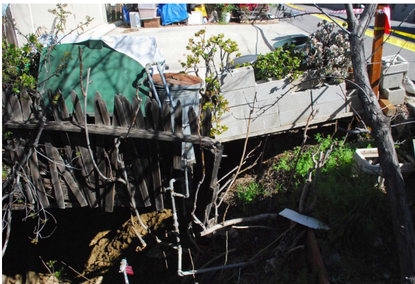
Figure 3.63 – Home in South Pasadena was undermined by a broken water main, was evacuated due to threat of imminent structural failure.
