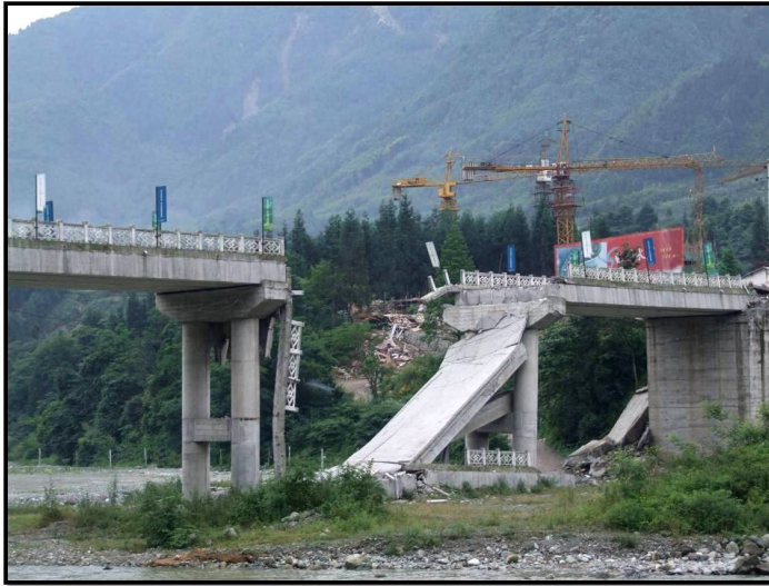
Figure 4.7 – Bridge span fallen from intermediate support. Taiwan. Photo courtesy Dave Swanson, EERI.
