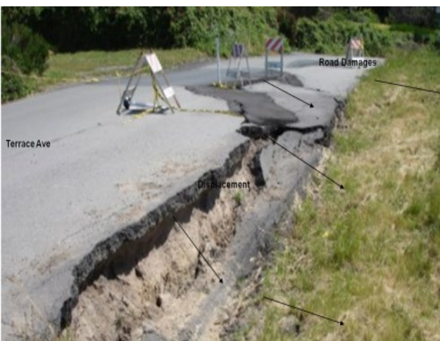
Figure 4.11 – Road scarp damage. Photo courtesy Cal OES.
