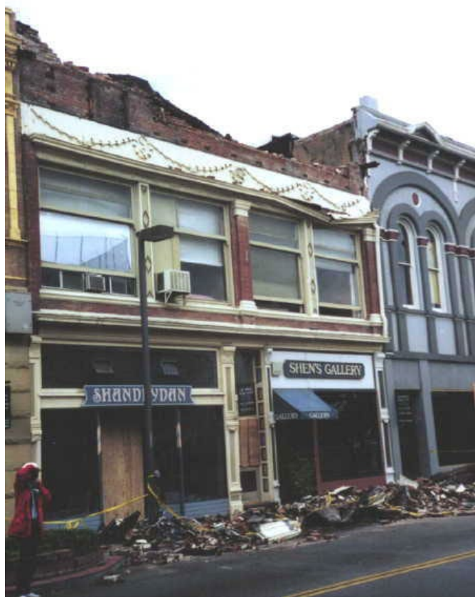
Figure 3.85 – Parapet failure in a historic building in downtown Santa Cruz, due to the 1989 Loma Prieta Earthquake.
