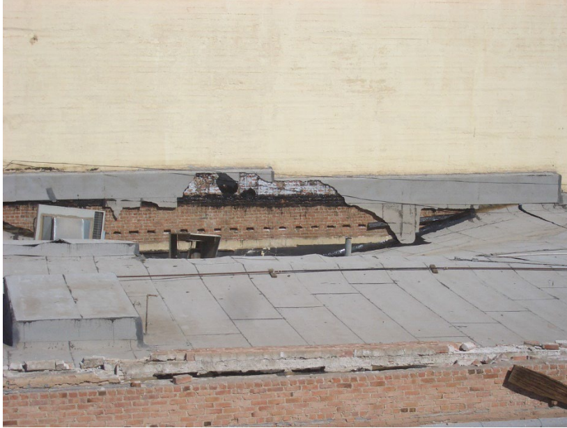
Figure 3.66 – Roof diaphragm pulled out from supports in brick wall during the 2010 Baja Earthquake. Photo courtesy David Karina.
