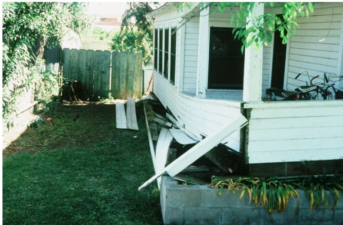
Figure 3.9 – House slid off its foundation, 1994 Northridge Earthquake.
