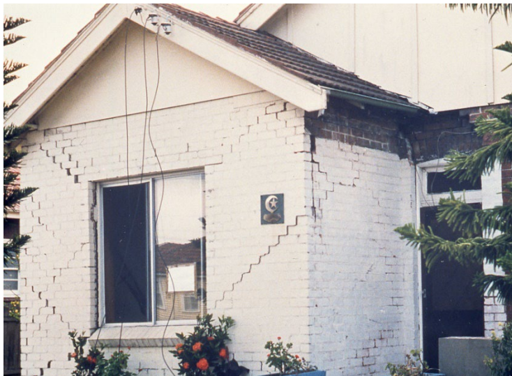
Figure 3.70 – Example of shear cracking in masonry wall house.
