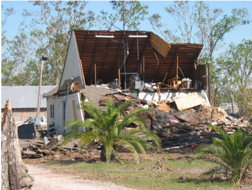
Figure 3.18 – Hurricane Katrina winds tore off the back of this house. Photo courtesy Raymond Lui.
