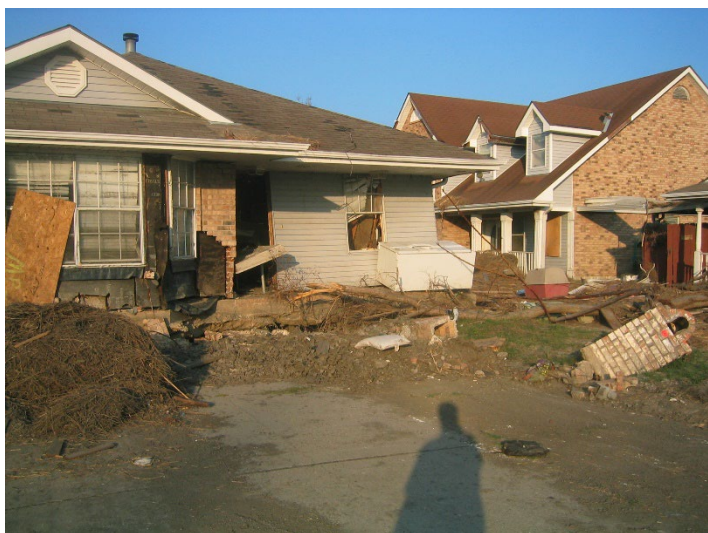
Figure 3.15 – Flooding 22 feet deep floated a home with a concrete post-tension slab right out of the ground. 2005 Hurricane Katrina. Photo courtesy Raymond Lui.
