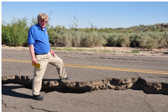
Figure 4.12 – Road damage due to the 2010 Baja Earthquake. Photo courtesy Fred Turner, EERI.
