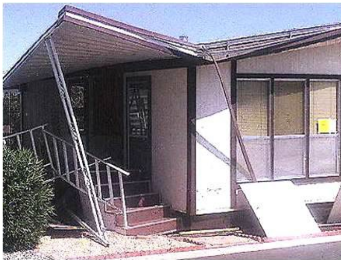
Figure 3.77 – Manufactured home collapsed on its supports. Stairs are now partway up in the door, and the side awning is unstable. Was tagged RESTRICTED USE, likely for possession retrieval.
