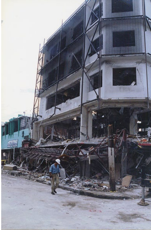
Figure 3.33 – Loss of an entire floor due to a natural gas explosion in the Humberto Building in Puerto Rico in 1996.
