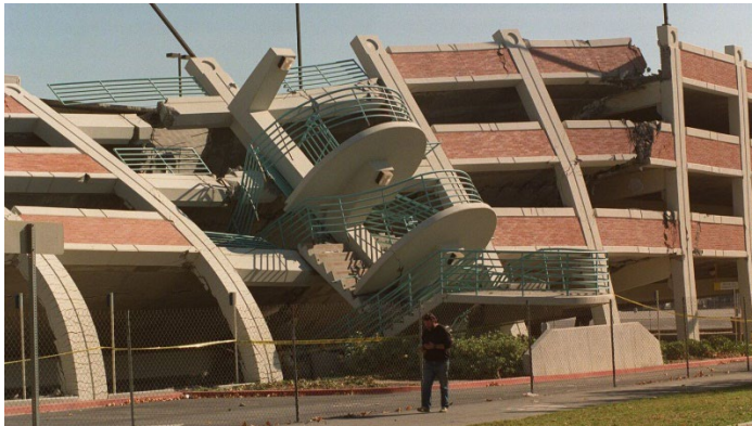
Figure 3.65 – Failed parking structure from the 1994 Northridge Earthquake.
