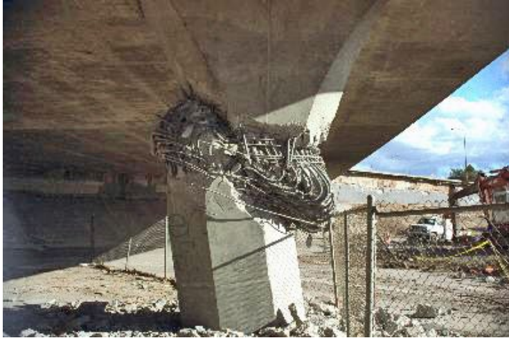
Figure 4.9 – Interstate 10 column collapse, 1994 Northridge Earthquake.
