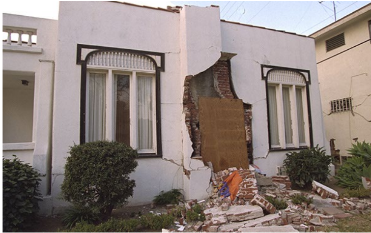
Figure 3.69 – Earthquake destroyed chimney.
