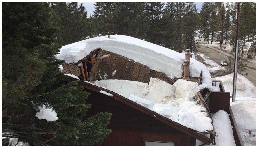
Figure 3.27 – Snow load caused full collapse of roof. 2023 South Tahoe Snow Load Damage. Photo courtesy Gurbir Singh.
