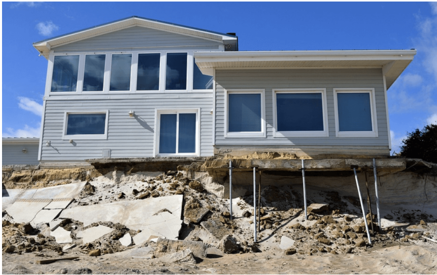
Figure 3.13 – Storm and flood erosion washed away supporting soils from under foundation. House is now UNSAFE.
