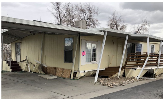
Figure 3.71 – Manufactured home damaged in an earthquake. Collapsed on foundation piers. Tagged UNSAFE.
