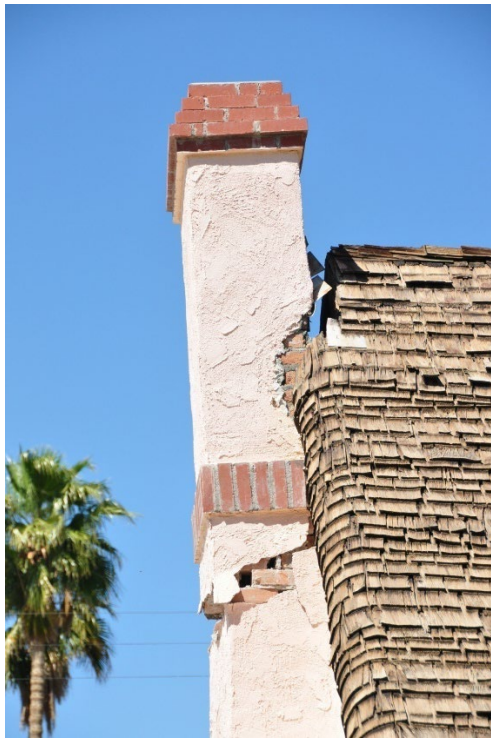
Figure 3.7 – Cracked chimney, 1994 Northridge Earthquake.
