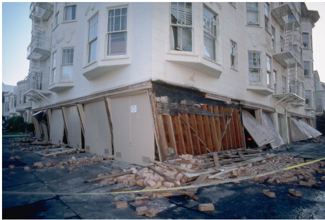
Figure 3.5 – Partial soft story failure, 1989 Loma Prieta Earthquake.
