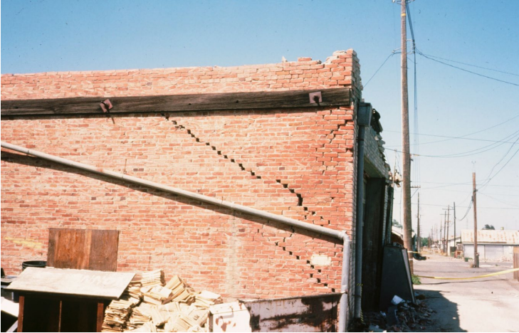
Figure 4.31 – Shear cracking in URM building. Photo courtesy Cal OES.
