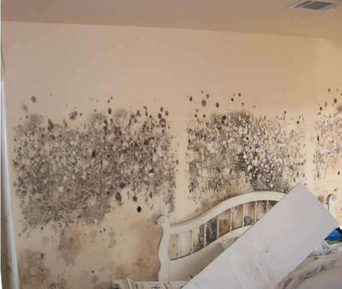
Figure 5.16 – Mold infestation after a flood disaster. Photo courtesy Raymond Lui, SEA.
