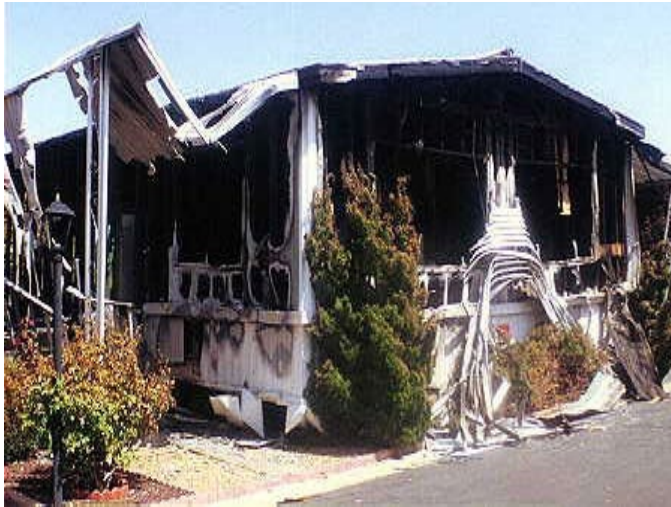
Figure 3.76 – Manufactured home was destroyed in a fire. Was tagged UNSAFE to keep people out of the dangerous conditions within.
