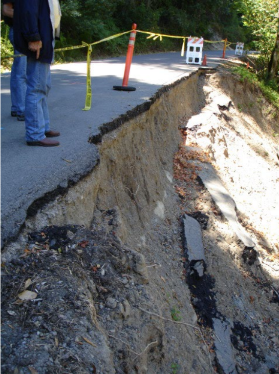
Figure 4.10 – Road slip out due to oversaturation of soil. Photo courtesy Cal OES.
