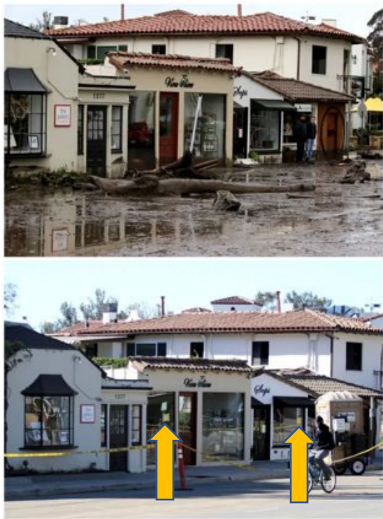
Figure 3.46 – 2018 flooding in Montecito, CA, before and after flooding. Buildings tagged RESTRICTED USE due to cleanup and mold abatement before occupancy is possible. Arrows in lower photo point to tags still in place weeks after cleanup began.
