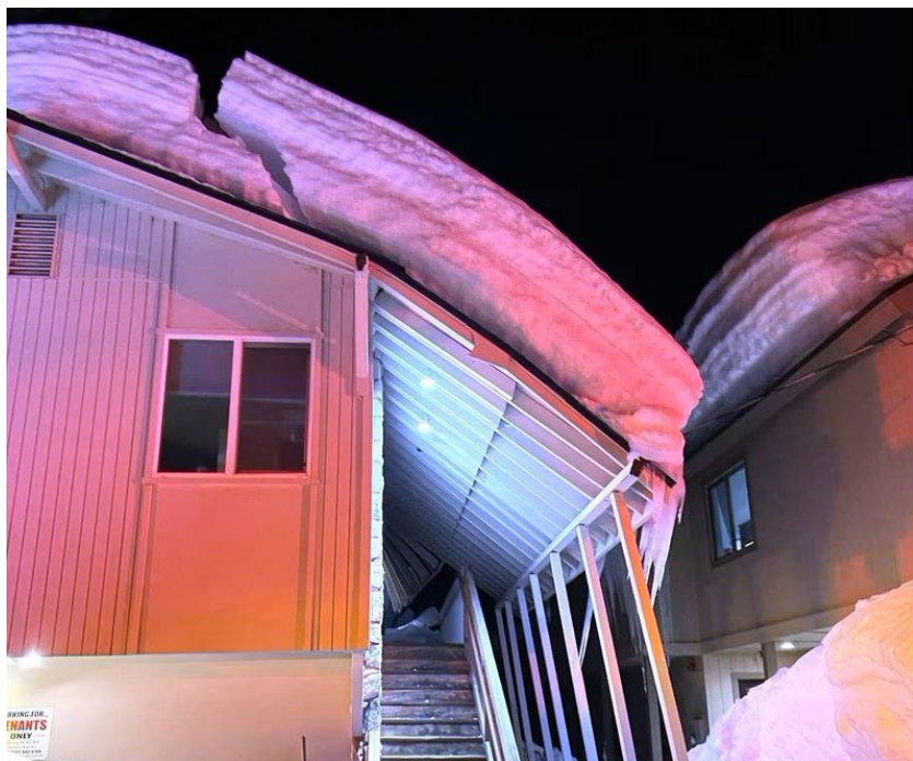
Figure 3.26 – Snow load caused failure of apartment roof and endangered structure, which was red-tagged. 2023 South Tahoe Snow Load Damage mission. Photo courtesy Gurbir Singh.
