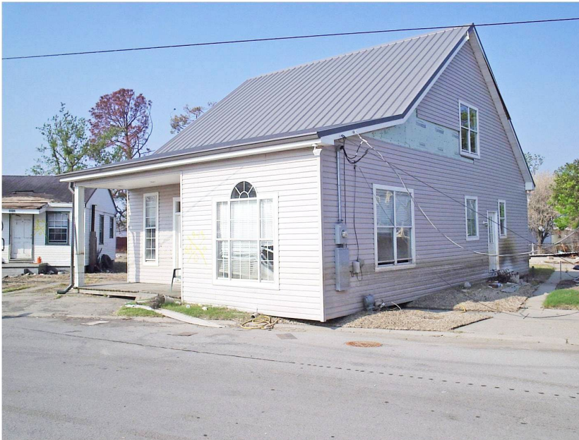
Figure 4.33 – House floated off foundation. Photo courtesy Raymond Lui.
