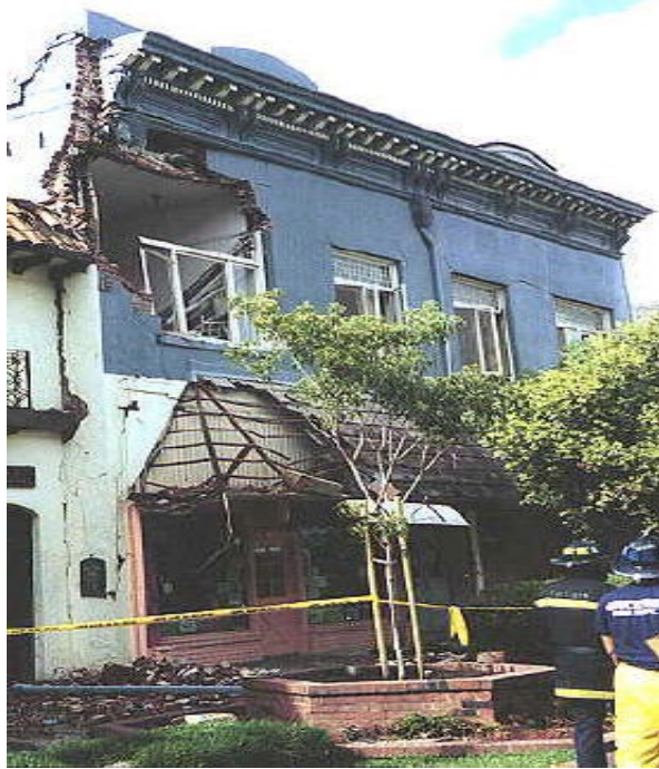
Figure 3.86 – Partial collapse of a brick wall in a historic building in downtown Santa Cruz due to the 1989 Loma Prieta Earthquake.
