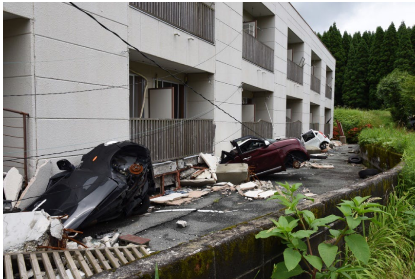
Figure 3.68 – Full collapse of soft story. Apartment building completely crushed the parking floor underneath it, including cars.
