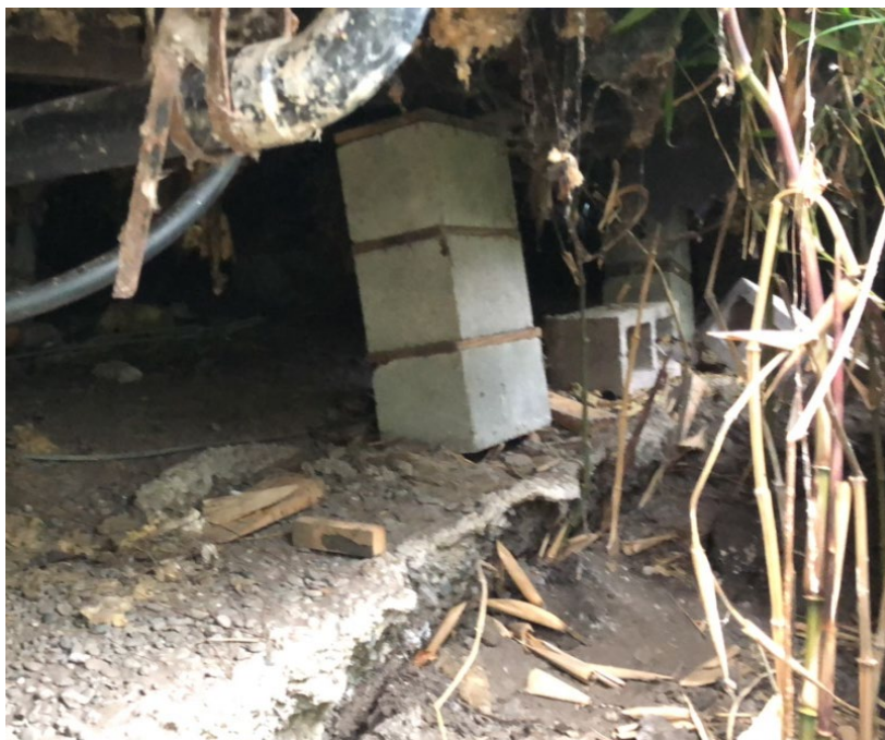
Figure 3.62 – Manufactured home shifted and twisted 4 inches off its foundation piers, which were rendered unstable. 2022 Ferndale Earthquake. Photos courtesy Gurbir Singh.
