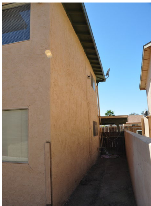
Figure 4.24 – Rigid end of apartment building shows no damage. Photo courtesy Fred Turner, EERI.
