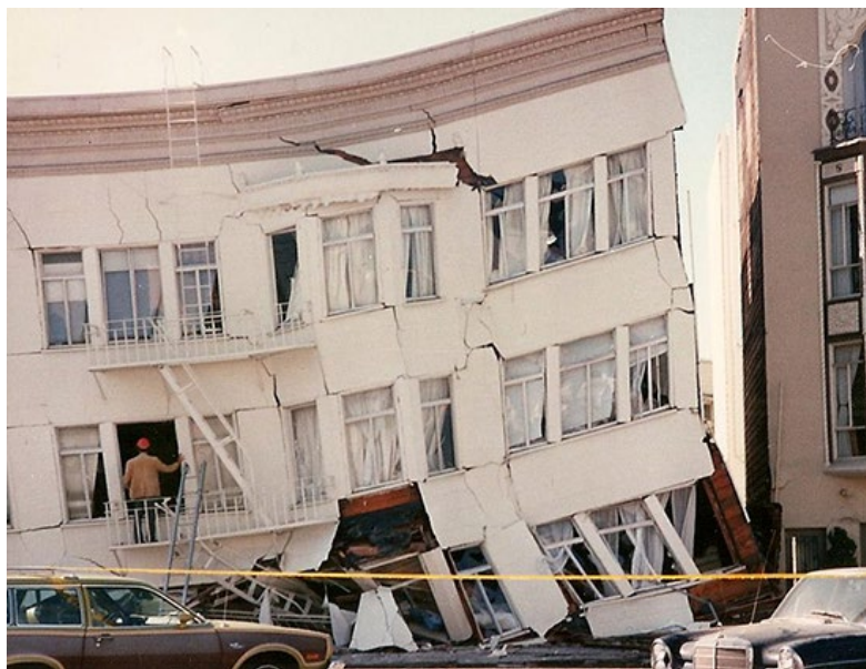
Figure 3.84 – Soft story failure in the San Francisco Marina District due to the 1989 Loma Prieta Earthquake.
