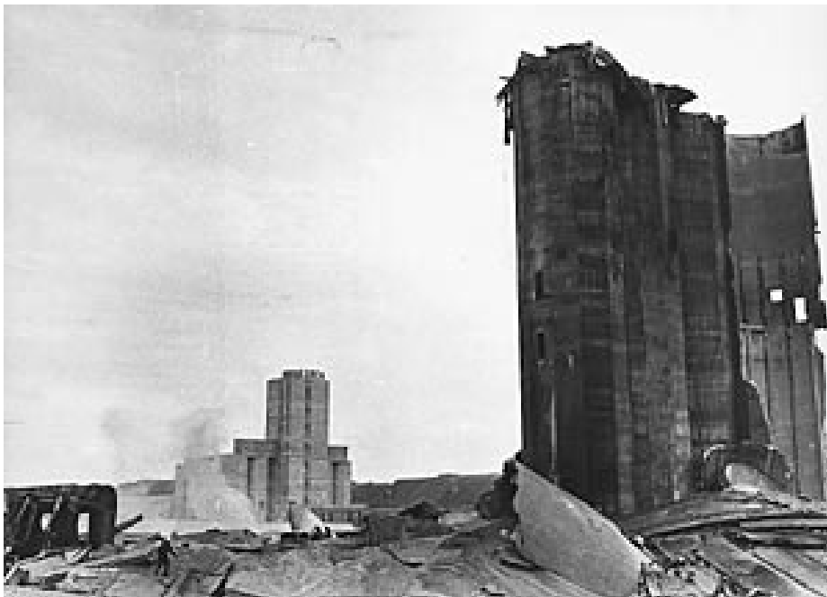
Figure 3.29 – Flour dust explosion destroyed a concrete granary. Fuels for dust explosions also include paper dust, wood dust, and some metal dusts.
