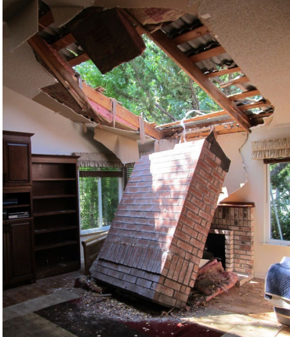
Figure 3.8 – Collapsed chimney through roof, 2014 Napa Earthquake.
