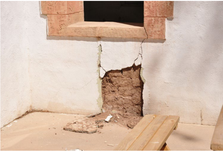
Figure 4.30 – Spalling of exterior stucco, showing adobe wall construction. Photo courtesy Fred Turner, EERI.
