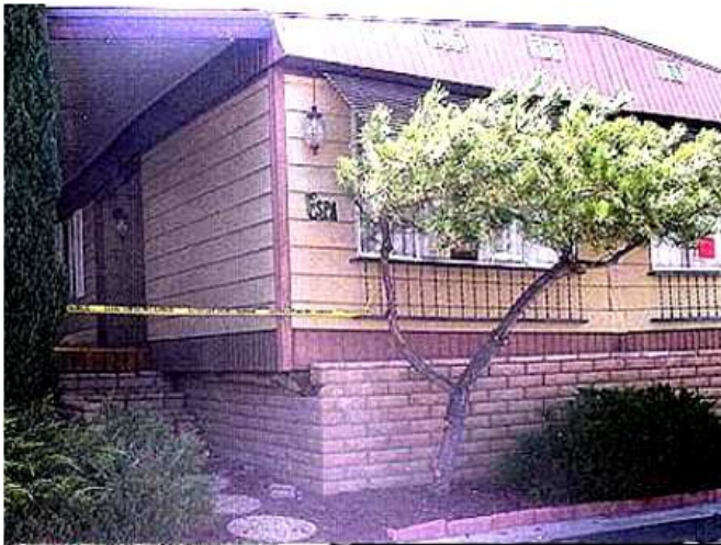
Figure 3.75 – This manufactured home was damaged in an earthquake. The steel frame shifted and is shown resting on the decorative but fragile brick skirting. The marriage line of this double-wide seems to be ready to pull apart at the bottom. Home was tagged UNSAFE and barricaded with caution tape.
