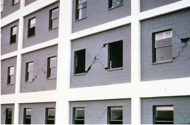
Figure 3.4 – Shear cracking in masonry infill wall.
