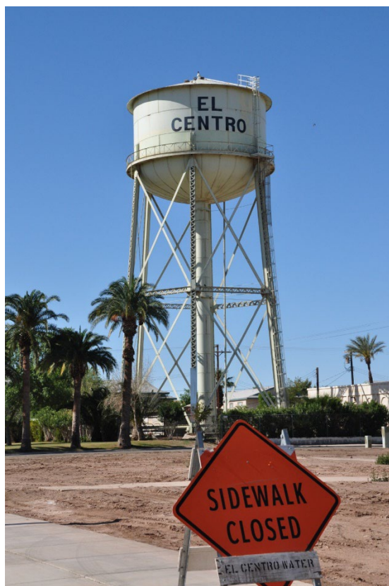
Figure 3.49 – El Centro Water Tower was 150 feet tall, and suffered extensive damage at its foundation supports due to base shear forces in the 2010 Baja Earthquake. Collapse zone was (150 \text{ ft} \times 1.5 =) 225 feet in radius. A duplex and an 8-unit apartment building were red-tagged as a result until the tower was removed. Photo courtesy David Karina.
