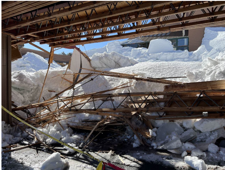
Figure 3.61 – Complete collapse of overhead structure due to snow load. 2023 Mono County Snow Load Mission. Photos courtesy Gurbir Singh.
