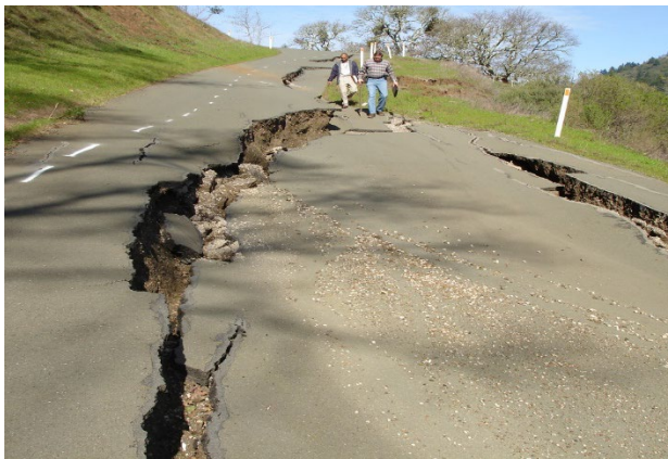
Figure 4.2 – This slope failure was caused by the “New Year’s Eve” storm of December 2005 through January 2006. Excessive soil saturation led to this failure condition called “block failure”, where the soil fails in large block sections.
