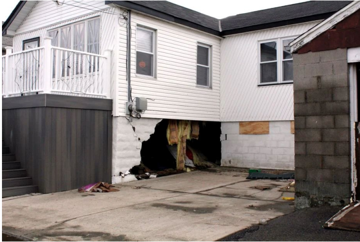
Figure 3.12 – Flood damage to foundation wall, 2012 Hurricane Sandy.
