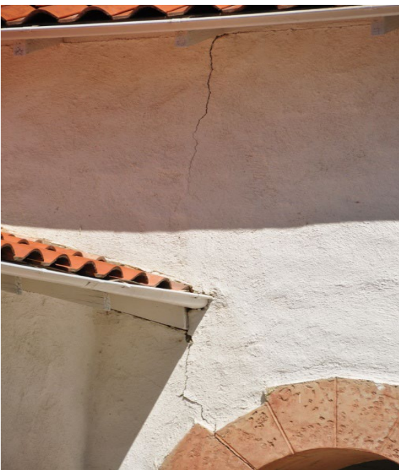
Figure 4.28 – Crack in wall over archway of adobe house. Photo courtesy Fred Turner, EERI.
