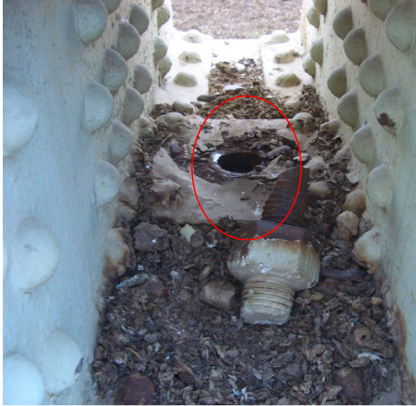
Figure 3.50 – Bolt at pad footing of the El Centro Water Tower was sheared off due to earthquake. Photo courtesy David Karina.
