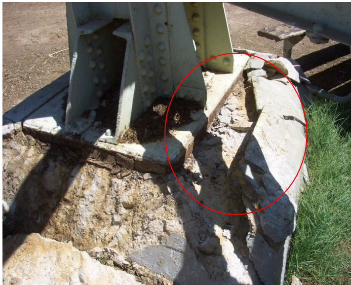
Figure 3.51 – Base plate movement at the El Centro Water Tower spalled the grout on the footing. Photo courtesy David Karina.
