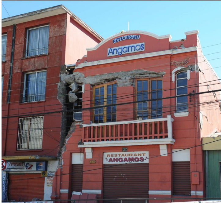
Figure 3.6 – Effects of seismic pounding, Chile.
