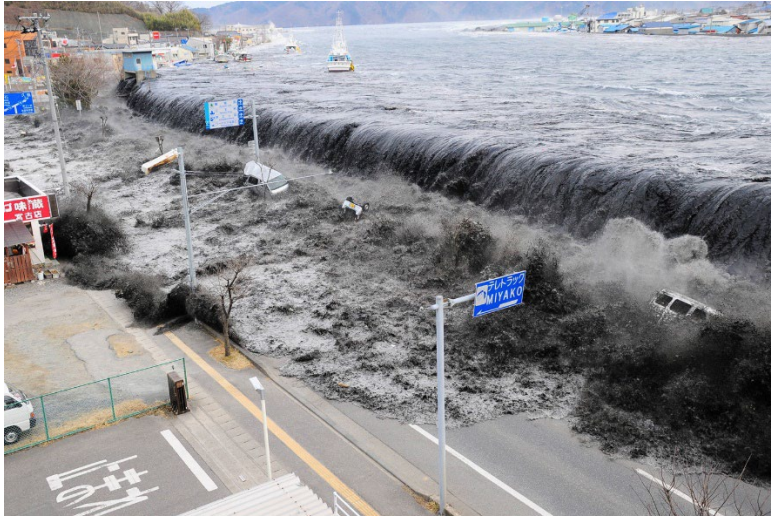
Figure 3.16 – The 2011 Tohoku Tsunami comes over the top of a 30-foot-high tsunami barrier wall.
