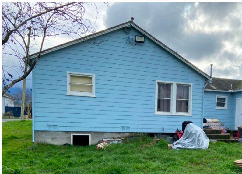
Figure 3.43 – House survived the 2023 Ferndale Earthquake. Minor drywall cracks and a minor crack in concrete foundation observed; could have been present before the earthquake. Tagged INSPECTED. Photo courtesy Gurbir Singh.
