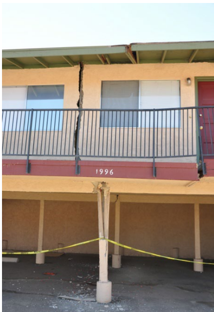
Figure 4.21 – Front view of damaged apartment building with soft story failure. Photo courtesy Fred Turner, EERI.
