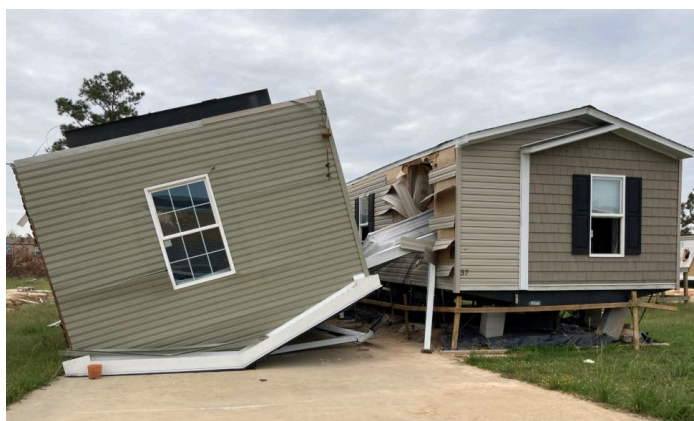
Figure 3.73 – A double-wide manufactured home split apart in a hurricane and a section rolled over.
