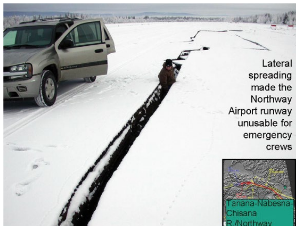
Figure 4.5 – Airport runway in Alaska rendered unusable due to lateral spreading caused by the 2002 Denali Earthquake. (Do not step into a crevasse, as this man has done!)
