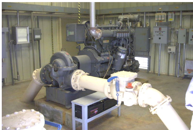
Figure 4.15 – Centrifugal pump with diesel motor.
