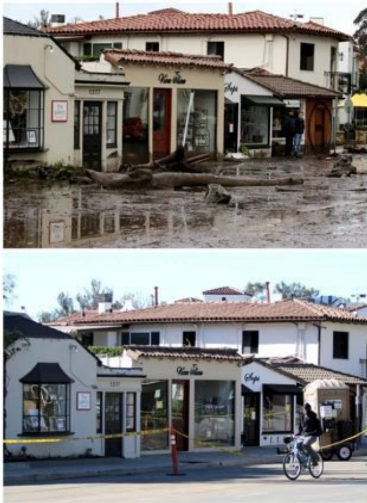
Figure 3.45 – 2018 flooding in Montecito, CA, before and after flooding. Buildings tagged RESTRICTED USE due to required cleanup and mold abatement prior to occupancy. Arrows in lower photo point to tags still in place weeks after cleanup began.
