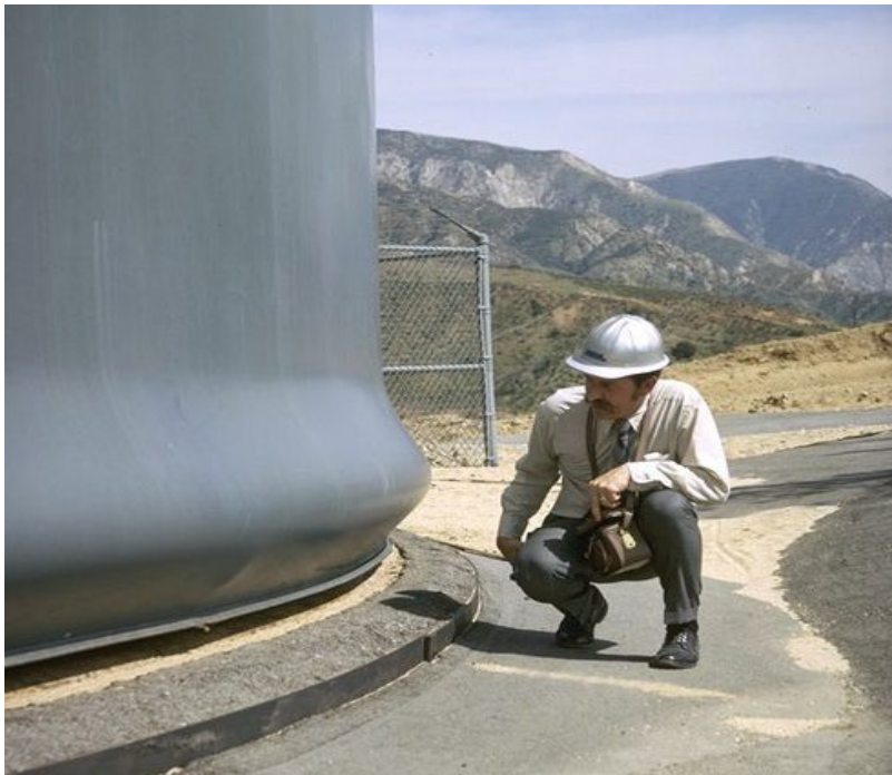
Figure 4.17 – Steel tank wall buckling, called 'elephant's foot,' caused by the tank structure failing while resisting seismic overturning forces.
