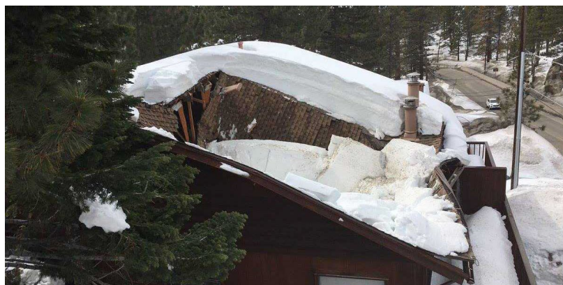
Figure 3.27 – Snow load caused full collapse of roof. 2023 South Tahoe Snow Load Damage. Photo courtesy Gurbir Singh.
