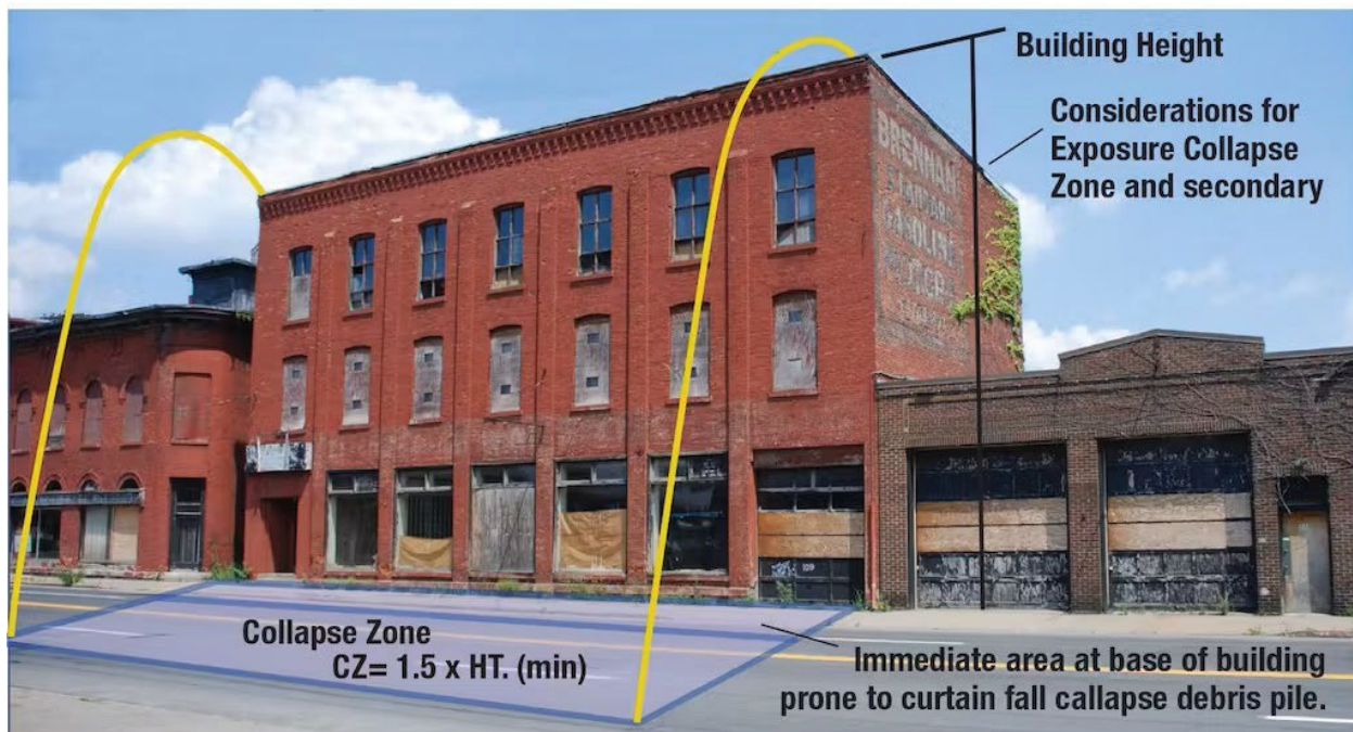
Figure 3.47 – Collapse zone illustration.
