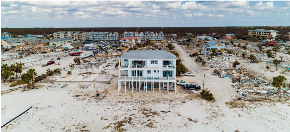
Figure 3.23 – The lone building in the foreground survived the 2018 Hurricane Michael winds and storm surge in the Florida panhandle, mostly due to being properly mitigated for flood and lateral wind loads.
