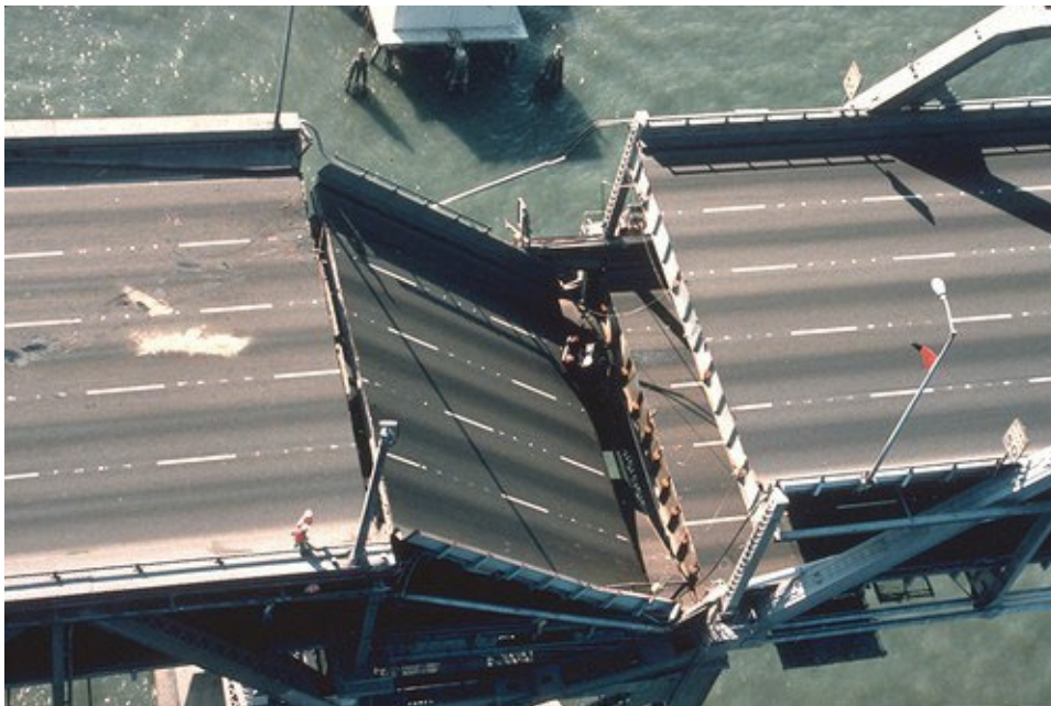
Figure 4.8 – Midspan bridge deck collapse, Bay Bridge, 1989 Loma Prieta Earthquake.
