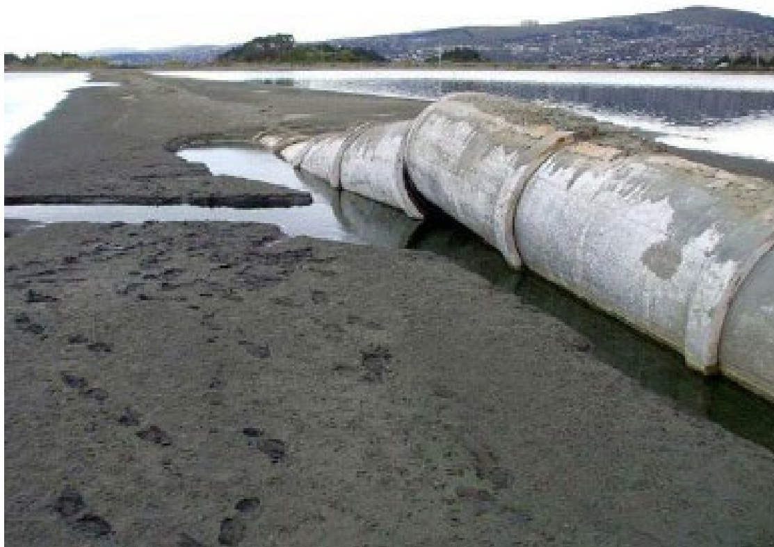
Figure 4.13 – Large asbestos-concrete (AC) pipe damaged by flotation and liquefaction. 2011 Canterbury Earthquake, New Zealand.
