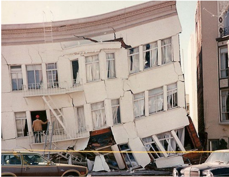
Figure 3.83 – Soft story failure in the San Francisco Marina District following the 1989 Loma Prieta Earthquake.
