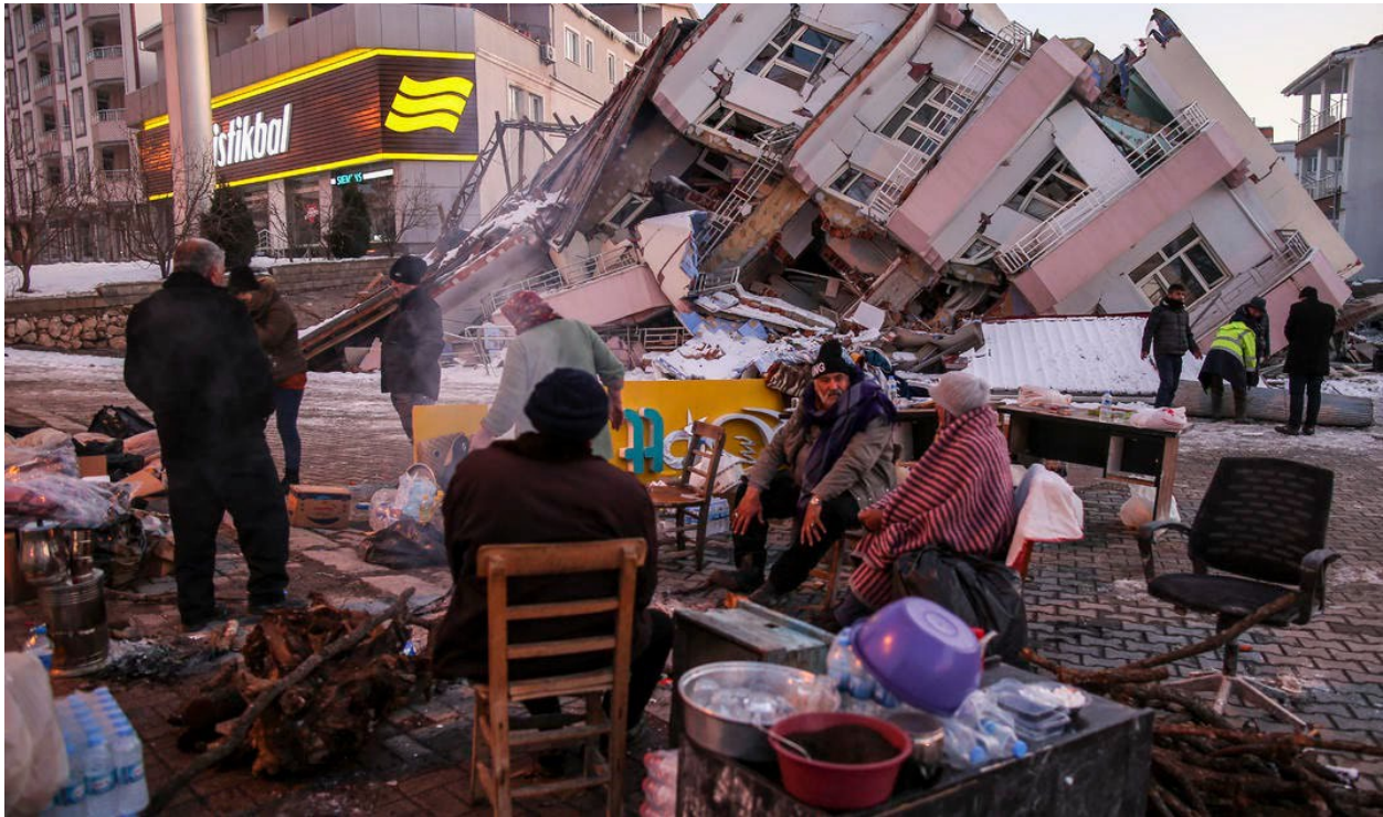
Figure 2.1 – Survivors wait outside a collapsed building.
