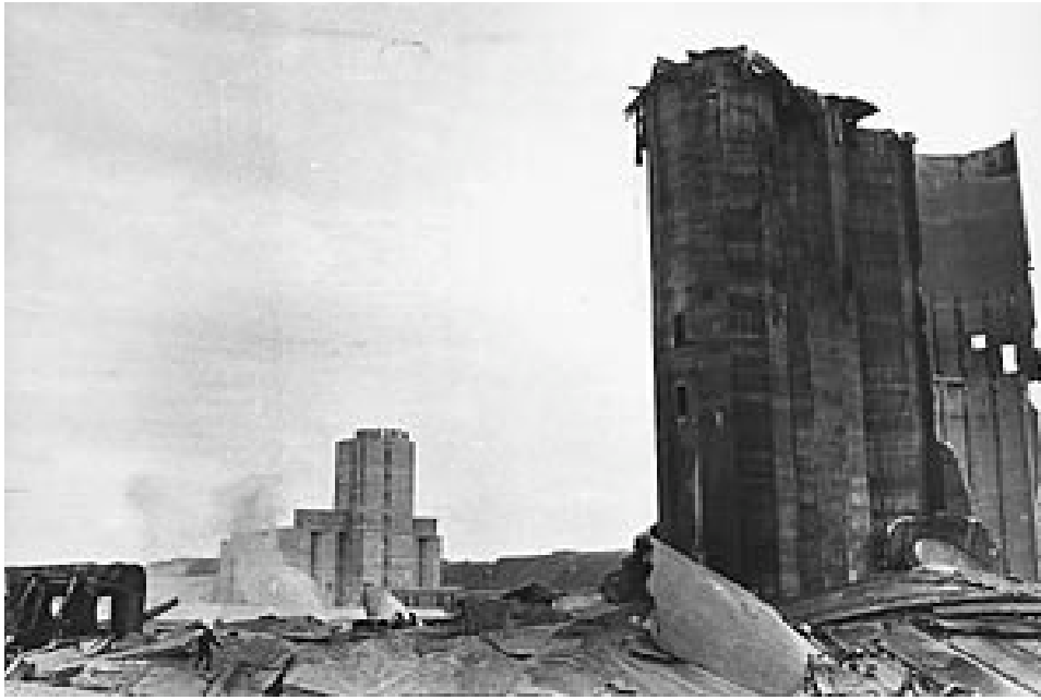
Figure 3.30 – Flour dust explosion destroyed a concrete granary. Fuels for dust explosions also include paper dust, wood dust, and some metal dust.
