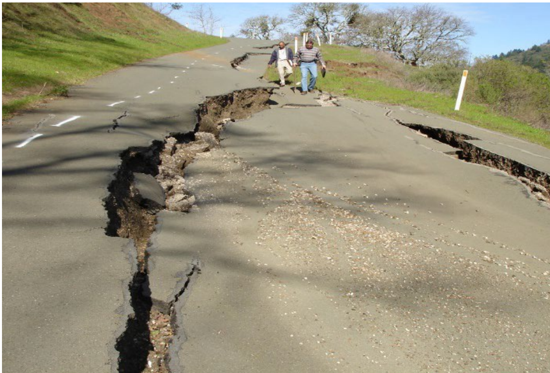
Figure 4.2 – This slope failure was caused by the “New Year's Eve” storm of December 2005 through January 2006. Excessive soil saturation led to this failure condition called “block failure”, where the soil fails in large block sections.
