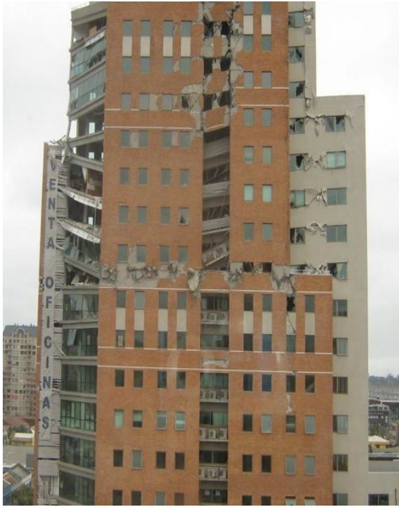
Figure 3.3 – Partial collapse of the O'Higgins Building in Concepcion, Chile.
