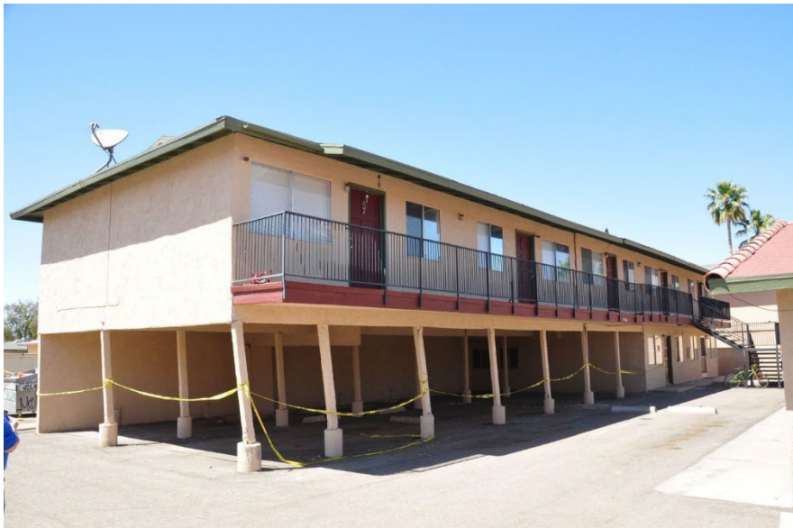
Figure 4.21 – Front view of damaged apartment building with soft story failure. Photo courtesy Fred Turner, EERI.
