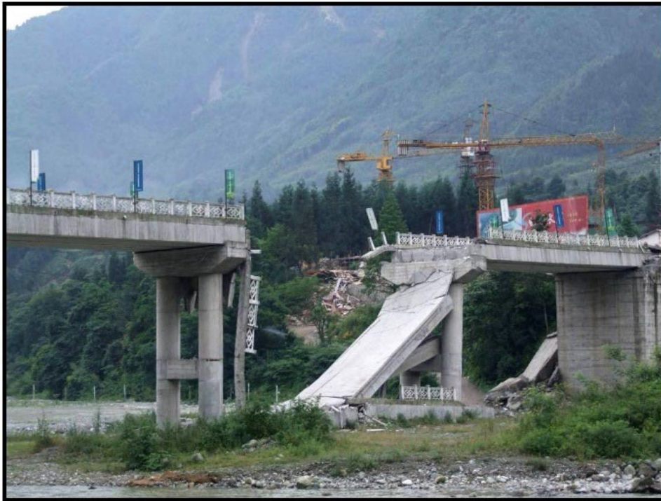
Figure 4.7 – Bridge span fallen from intermediate support. Taiwan. Photo courtesy Dave Swanson, EERI.
