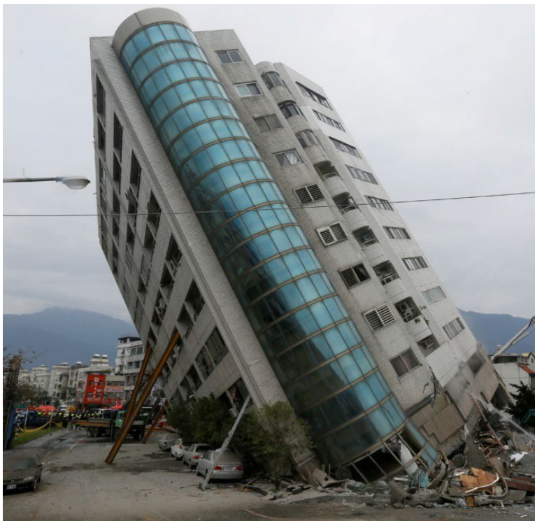
Figure 3.2 – Soft story failure, building severely tilting, 2018 Taiwan Earthquake.
