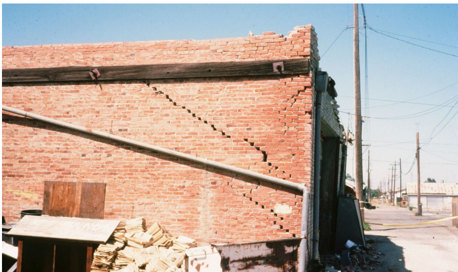
Figure 4.31 – Shear cracking in URM building. Photo courtesy Cal OES.
