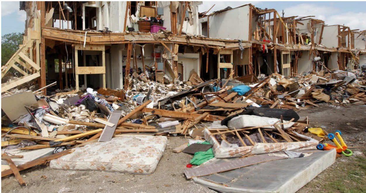
Figure 3.36 – Explosion damage to an apartment building in West, Texas (2013). Explosion originated at a local fertilizer plant.
