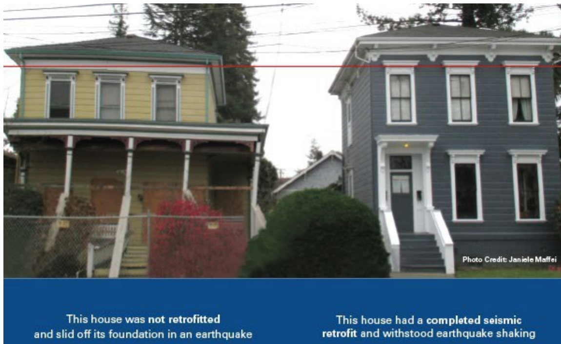
Figure 3.66 – Example of two homes side by side; left house had no seismic retrofit work and suffered damage, while the right house was completely retrofitted and suffered no damage.
