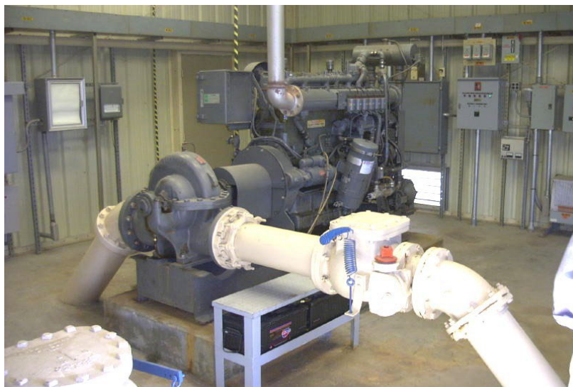
Figure 4.15 – Centrifugal pump with diesel motor.
