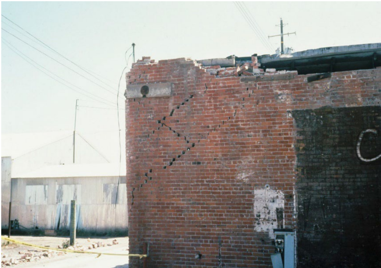
Figure 4.32 – Shear cracking in URM building. Photo courtesy Cal OES.
