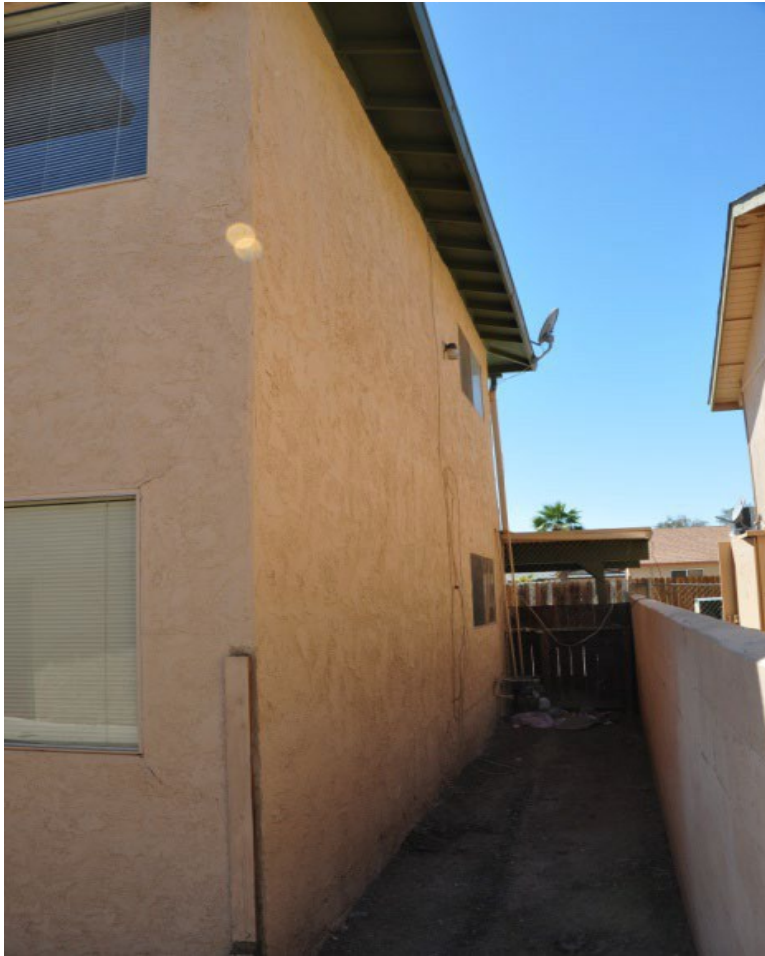
Figure 4.24 – Rigid end of apartment building shows no damage. Photo courtesy Fred Turner, EERI.
