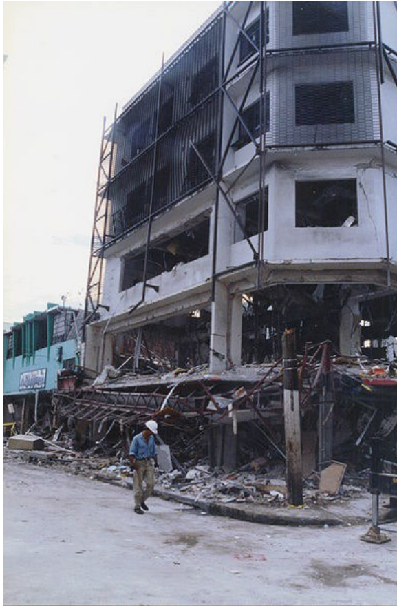
Figure 3.34 – Loss of an entire floor due to a natural gas explosion in the Humberto Building in Puerto Rico (1996).
