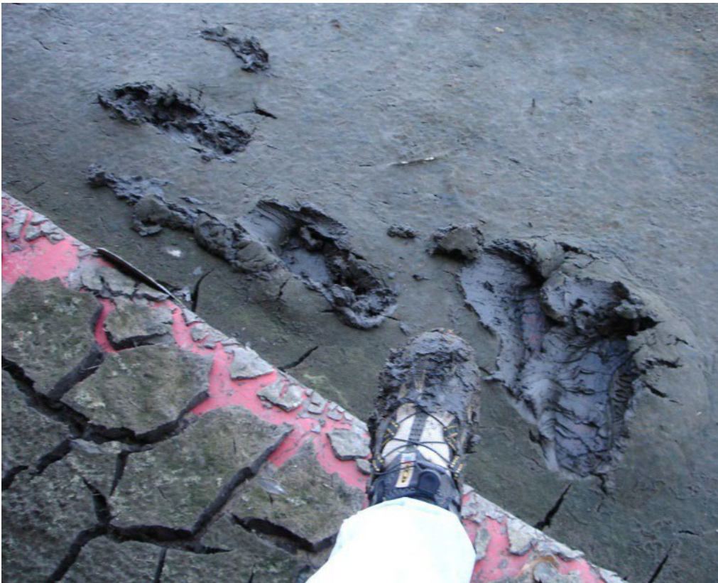
Figure 5.17 – Deep mud in street can be a slip or other safety hazard. Photo courtesy Raymond Lui, SEA.
