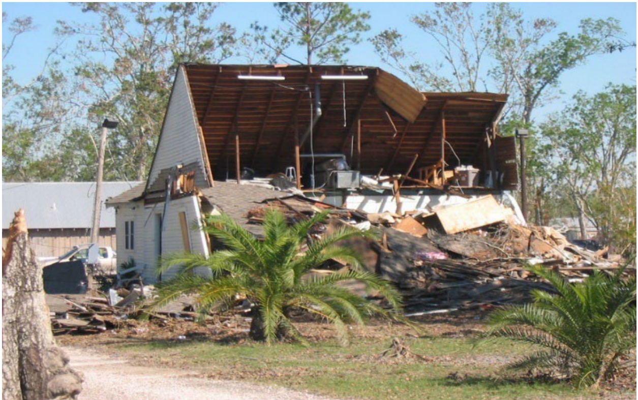
Figure 3.18 – Hurricane Katrina winds tore off the back of this house. Photo courtesy Raymond Lui.
