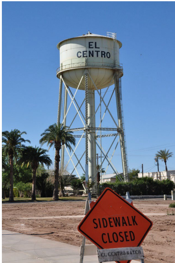
Figure 3.48 – El Centro Water Tower was 150 feet tall, and suffered extensive damage at its foundation supports during the 2010 Baja Earthquake. Collapse zone was (150 \text{ ft} \times 1.5 =) 225 feet in radius. A duplex and an 8-unit apartment building were red-tagged as a result until the tower was removed. Photo courtesy David Karina.
