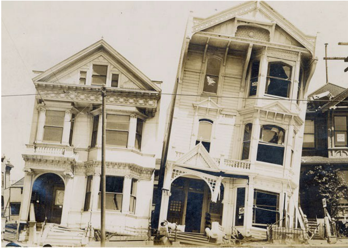
Figure 3.81 – Liquefaction causes tilting of these Victorian homes.
