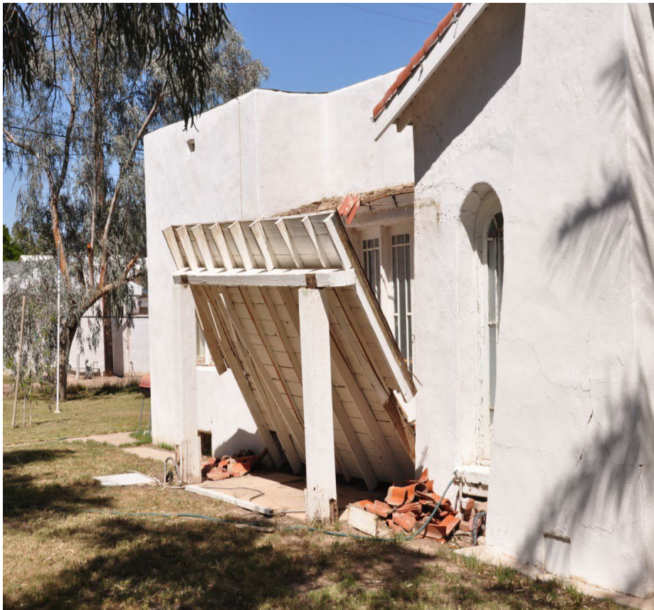
Figure 4.26 – Collapsed porch awning. Photo courtesy Fred Turner, EERI.
