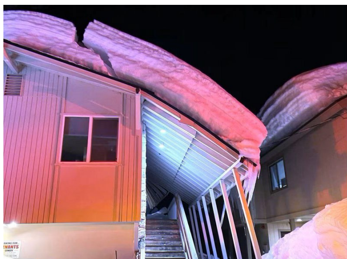
Figure 3.26 – Snow load caused failure of apartment roof and endangered structure, which was red-tagged. 2023 South Tahoe Snow Load Damage mission. Photo courtesy Gurbir Singh.
