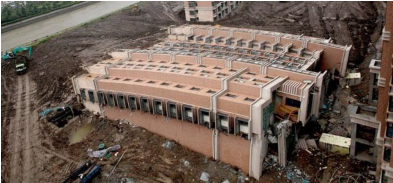
Figure 3.46 – Collapsed high-rise building in Taiwan after an earthquake.
