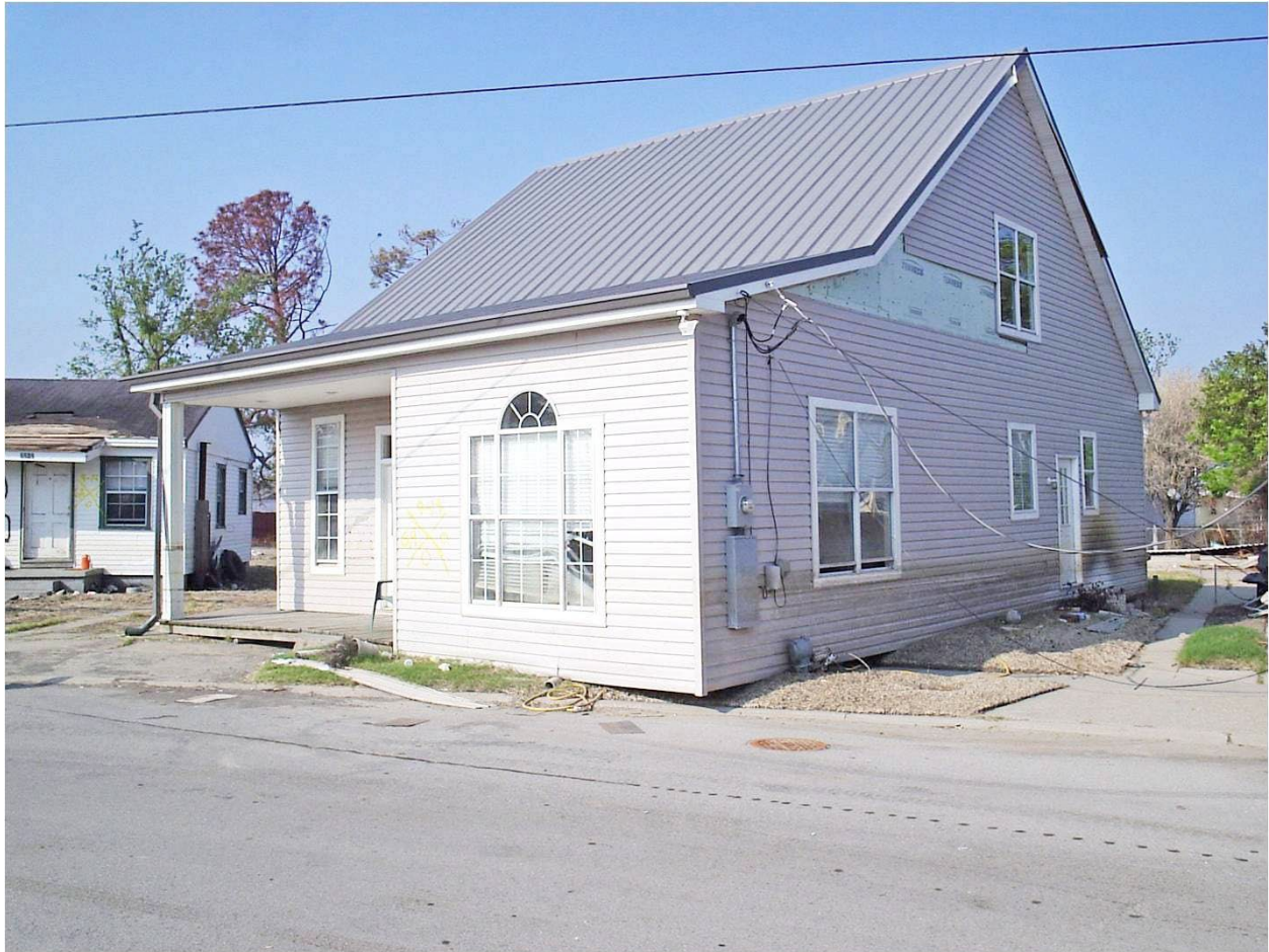
Figure 4.33 – House floated off foundation. Photo courtesy Raymond Lui.
