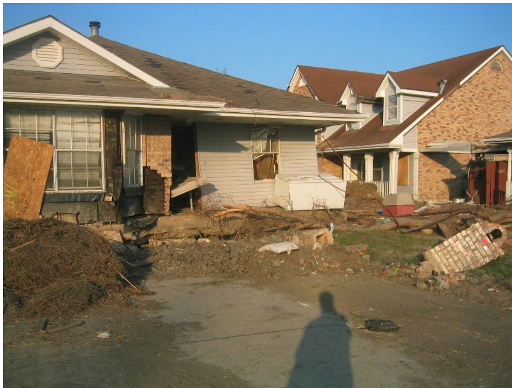
Figure 3.15 – Flooding, 22 feet deep floated a home right off its concrete post-tension slab. 2005 Hurricane Katrina. Photo courtesy Raymond Lui.
