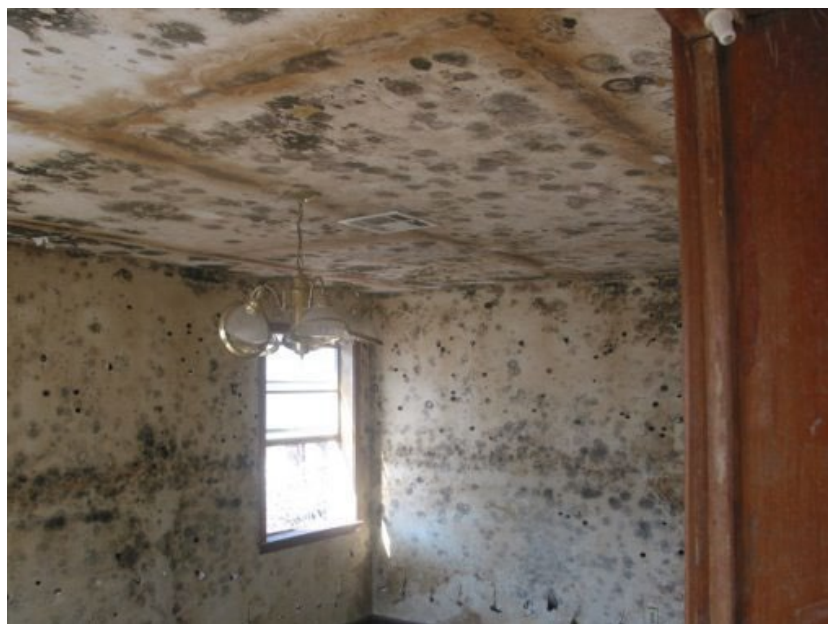
Figure 3.11 – Mold impacting residence, 2005 Hurricane Katrina. Photo courtesy Raymond Lui.
