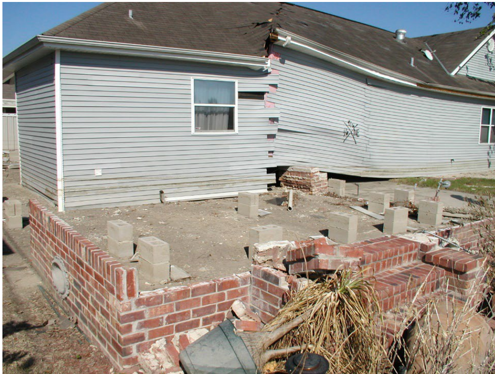
Figure 3.14 – House floated off its foundation and came to rest destructively on a different foundation. 2005 Hurricane Katrina. Photo courtesy Raymond Lui.
