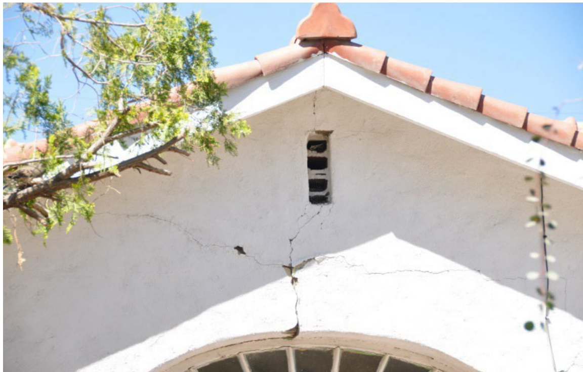
Figure 4.29 – Crack in wall over archway of adobe house. Photo courtesy Fred Turner, EERI.
