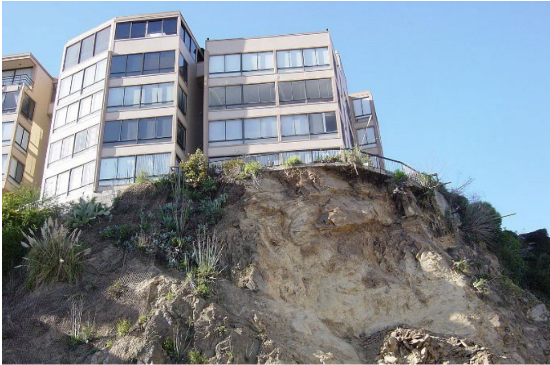
Figure 4.1 – Head scrap of a 2008 rockslide in San Francisco is far enough away from the mid-rise towers so as not to be an imminent threat.
