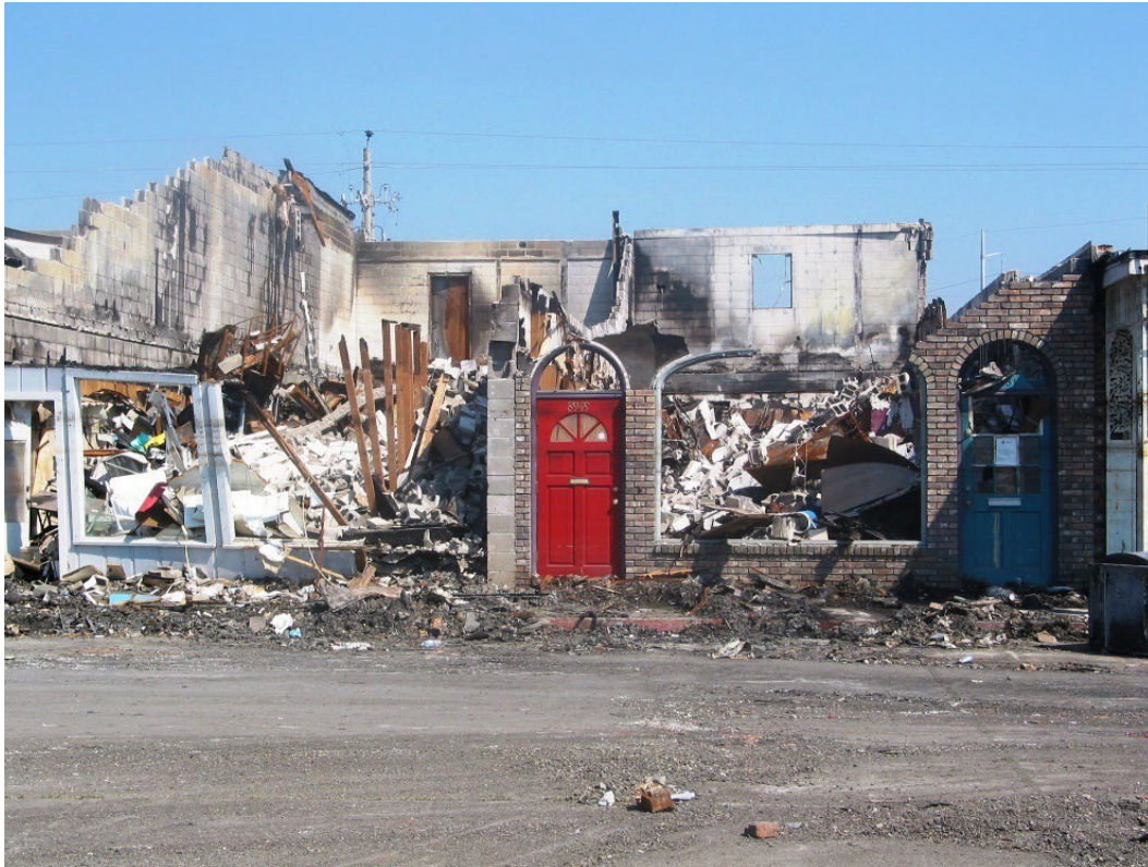
Figure 3.21 – Hurricane Katrina tore the roof off this building and damaged the unreinforced masonry walls. Subsequent storm surge flooding filled the building to about seven feet above the ground, and the part of the building above the water line caught on fire. This photo shows that the door is still intact. Photo courtesy Raymond Lui.
