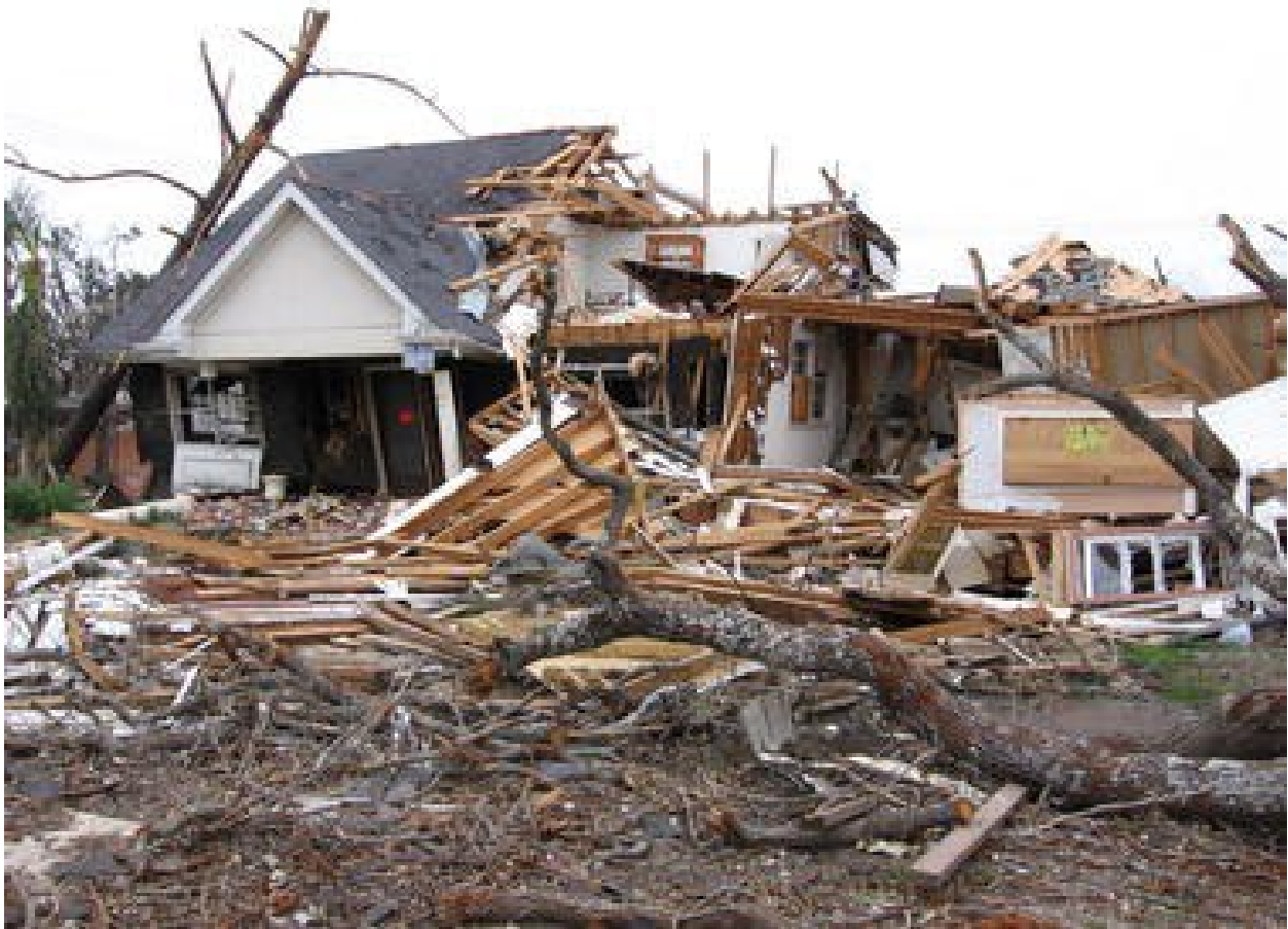
Figure 3.63 – House heavily damaged by 2005 Hurricane Katrina.
