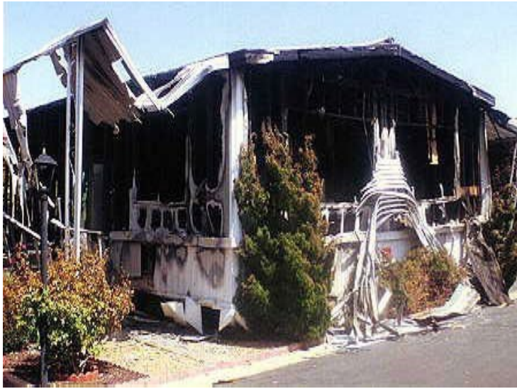
Figure 3.75 – Manufactured home was destroyed in a fire. The remnants were tagged UNSAFE to keep people out of the dangerous conditions within.
