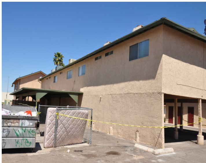
Figure 4.23 – Slight rotation out of plane along back of apartment building. Photo courtesy Fred Turner, EERI.
