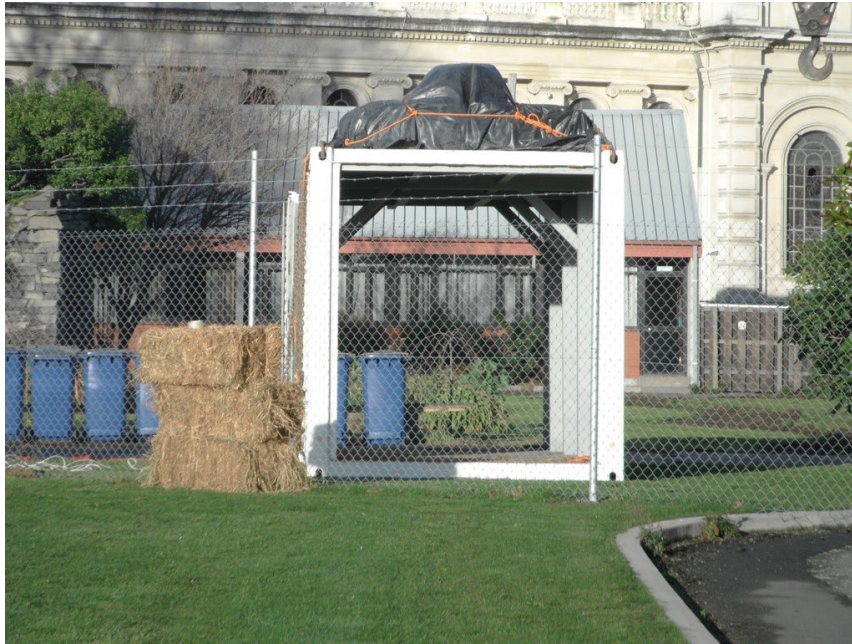
Figure 2-17: Shipping container retrofitted to serve as a debris shed. Christchurch, New Zealand.
