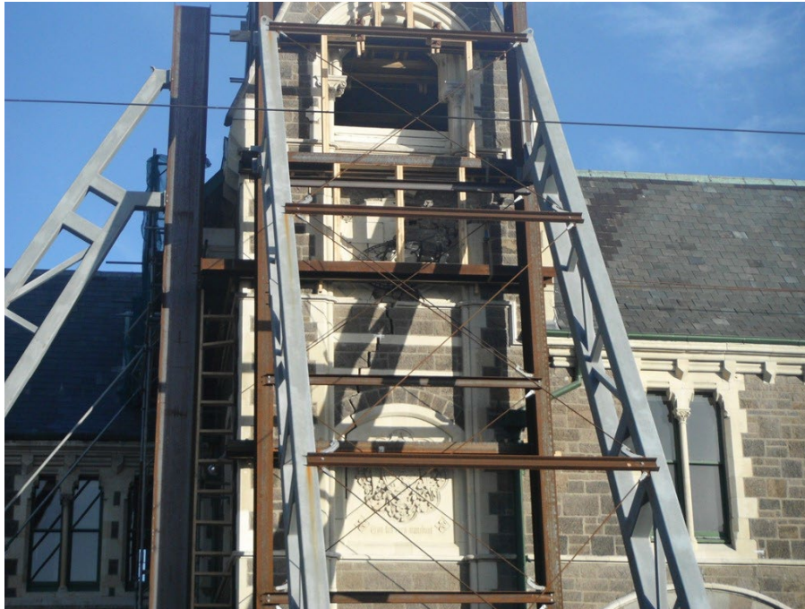
Figure 2-19: Steel shoring, Christchurch, New Zealand.
