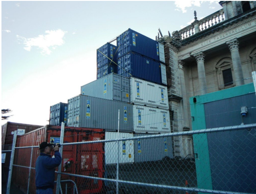
Figure 2-20: Shipping containers used to shore up masonry building in Christchurch, New Zealand.
