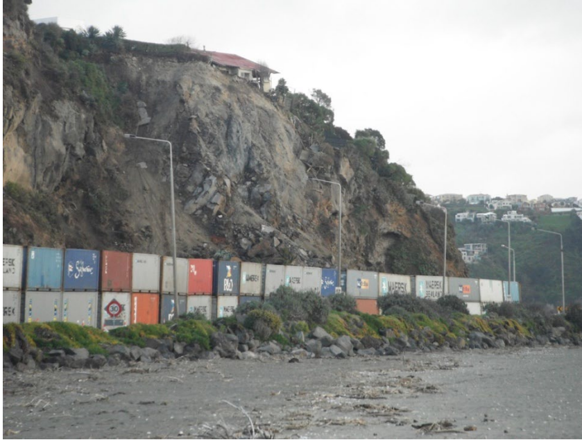
Figure 2-16: Containers used to protect coastal highway from rock falls, New Zealand.
