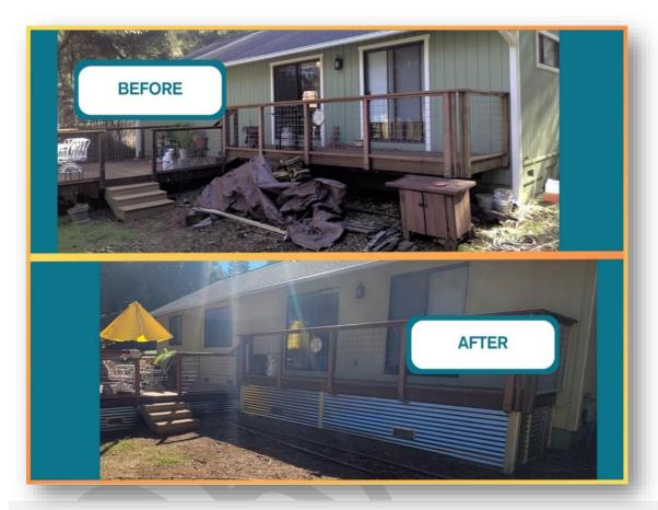
This image shows a deck that has undergone home hardening retrofits. The space around the deck was cleared of miscellaneous flammable materials and the underside of the deck was fully enclosed. Enclosing the deck prevents flammable materials from accumulating below the deck and prevents flames and embers from igniting the deck from below.
