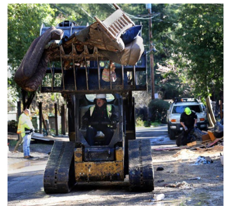
Curbside debris collection after the 2019 Russian River Flooding (Sonoma)
