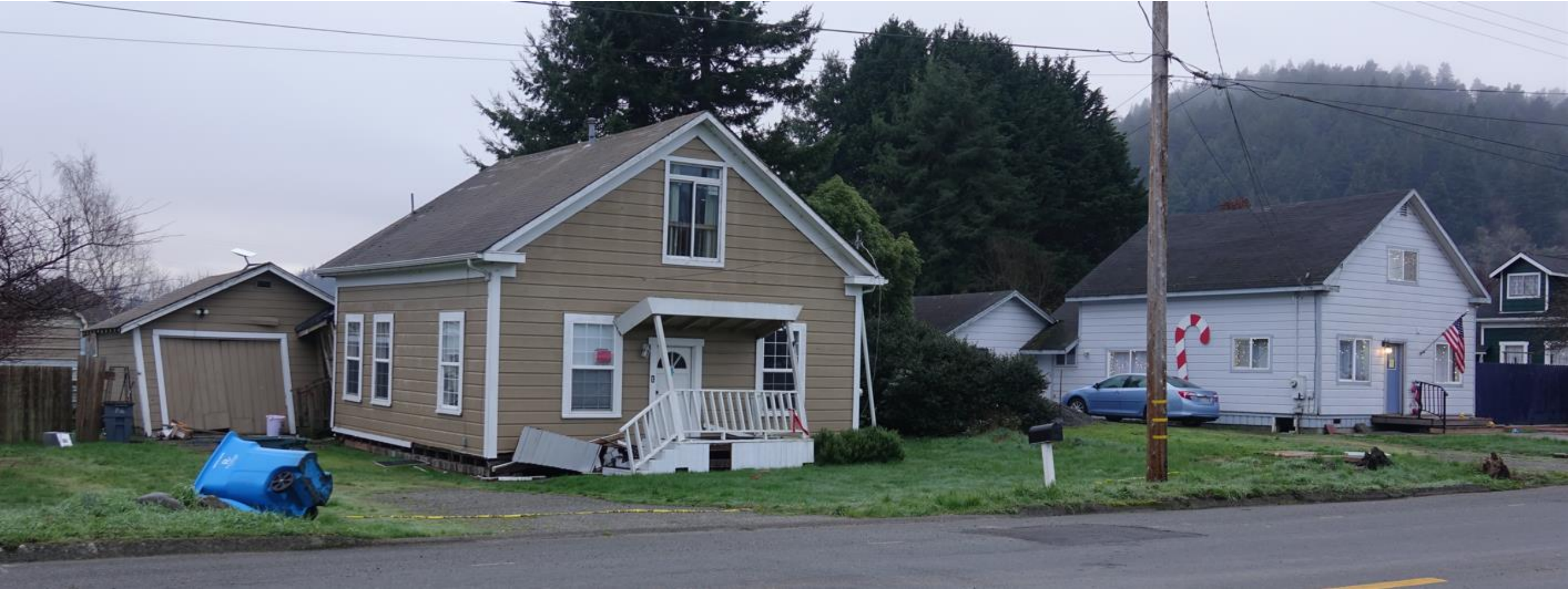
Unretrofitted – Red Tagged
