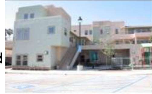
Camino Gonzalez Farmworker Family Apartments Oxnard CA
