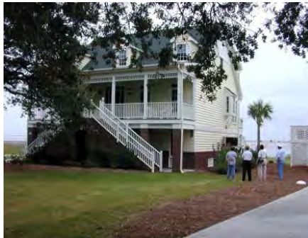
Mitigation: Elevating a home by the river
