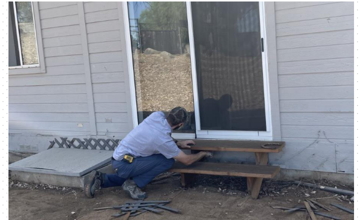
Removing the Combustible Skirting
