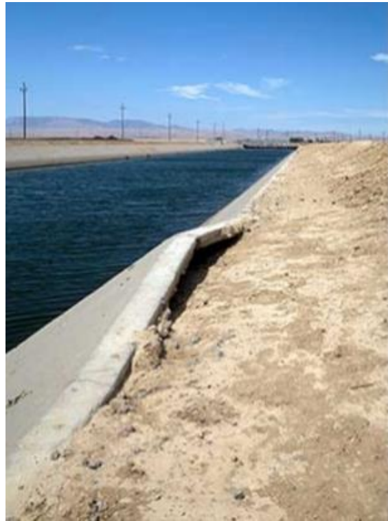
Figure 18-1. Physical Signs of Subsidence
