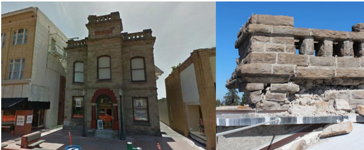
Source: South Napa Earthquake SMART Assessment Report 2014
