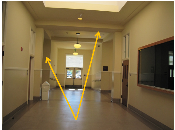
Tube steel frames were installed on both sides of the central hallway and along exterior walls. Frames were connected by steel cross members. (Photo: Bonnie Hanchett)
