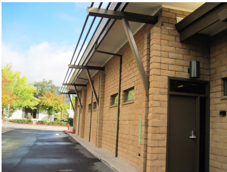
Steel beams along with vertical bracing were added to support roof overhang. (Photo: Bonnie Hanchett)
