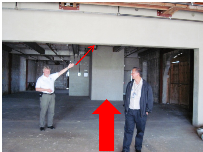
Mike Mahoney, Hazard Mitigation Engineering and Architecture Specialist points to reinforced concrete beam on first floor which was added for support as Emile Wong, Hazard Mitigation Engineer, looks on. The side of the concrete elevator is visible in the background. (Photo: Bonnie Hanchett)
