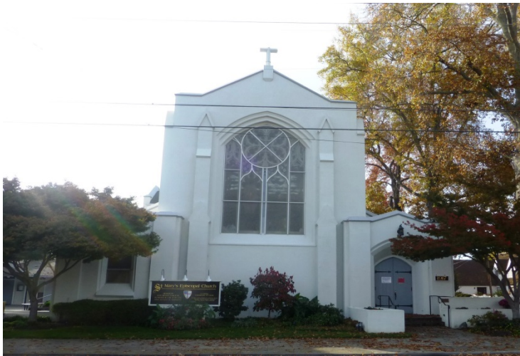
St. Mary's Episcopal Church, in Napa, CA, was seismically retrofitted in 1999. (Photo: Emile Wong)
