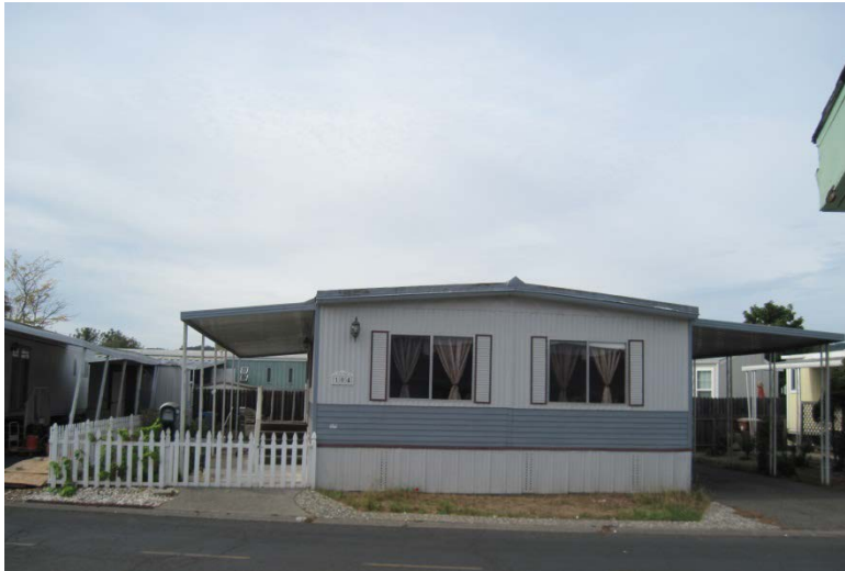
Karen Gibson's retrofitted mobile home remained virtually unscathed following a 6.0 magnitude earthquake in Napa County in 2014. (Photo: Bonnie Hanchett)
