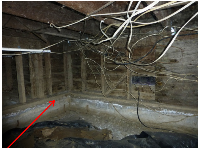
The sill plate is resting directly on top of the foundation and is secured with anchor bolts. (Photo: Emile Wong)
