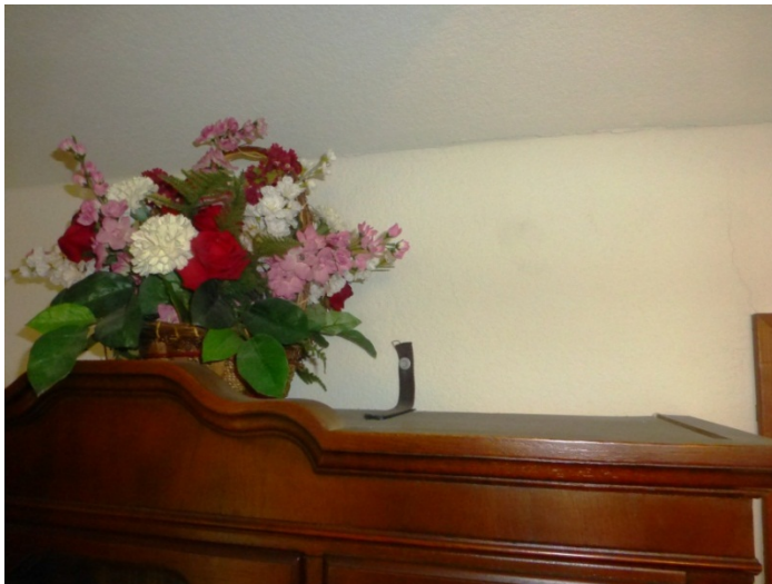
The china cabinet is in two pieces. The top and bottom were bolted together as a single unit and the top of the cabinet was anchored to the wall using two strappings. (Photo: Emile Wong)
