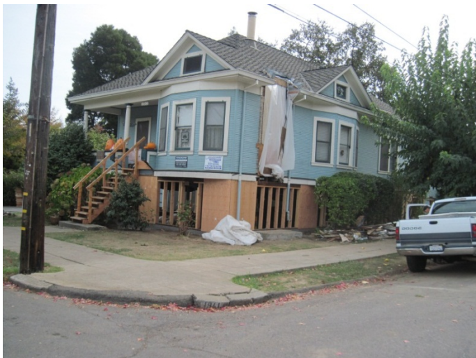
Repairs are on the way on an un-retrofitted home which suffered cripple wall failure. (Photo: Bonnie Hanchett)
