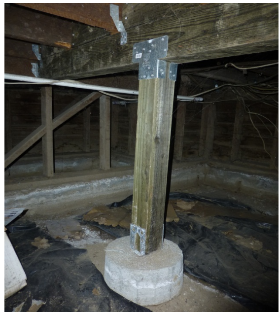
Additional wooden girders and posts were used to support the interior floor joists. (Photo: Emile Wong)
