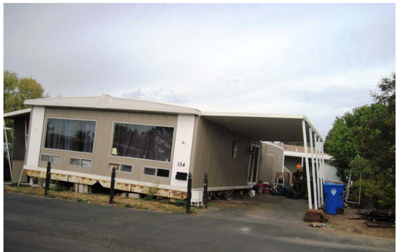
The 6.0 magnitude earthquake caused severe damage to a mobile home that was not seismically retrofitted. (Photo: Bonnie Hanchett)
