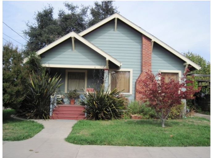
The 6.0 magnitude earthquake claimed only the chimney's top on this seismically retrofitted home (Photo: Bonnie Hanchett)
