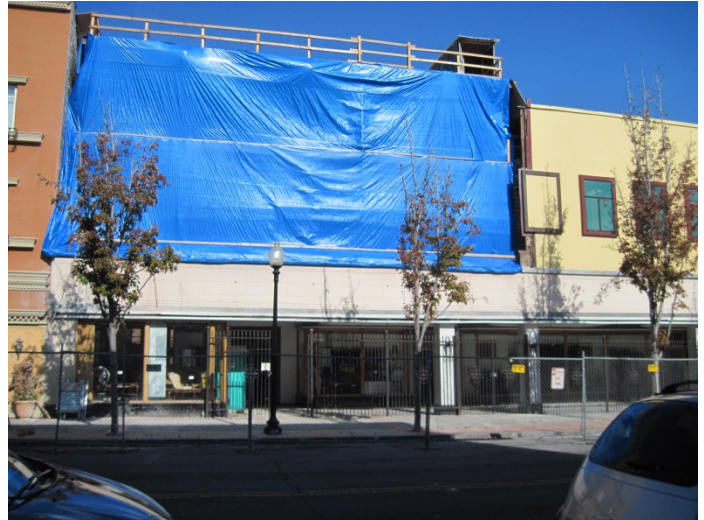
The un-retrofitted Raymond Building suffered damage to its roof and front facade along with interior damages. (Photo: Emile Wong)
