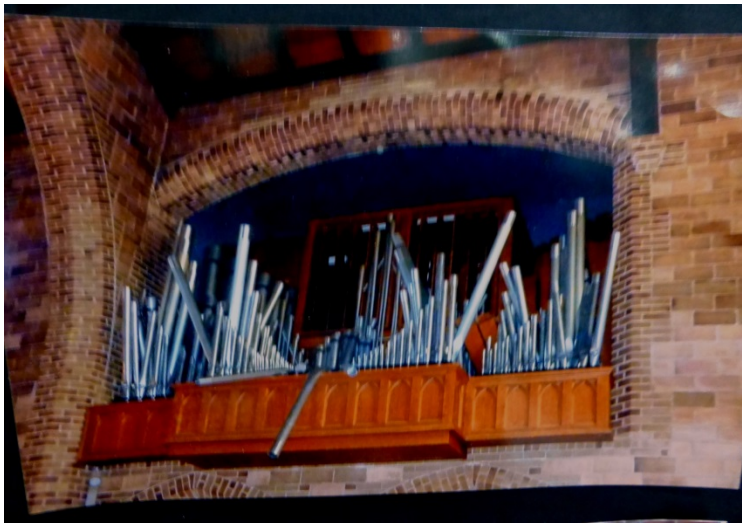
The pipe organ at St. Mary's Episcopal Church was damaged from the South Napa Earthquake, which occurred Aug. 24, 2014. (Photo: Emile Wong)
