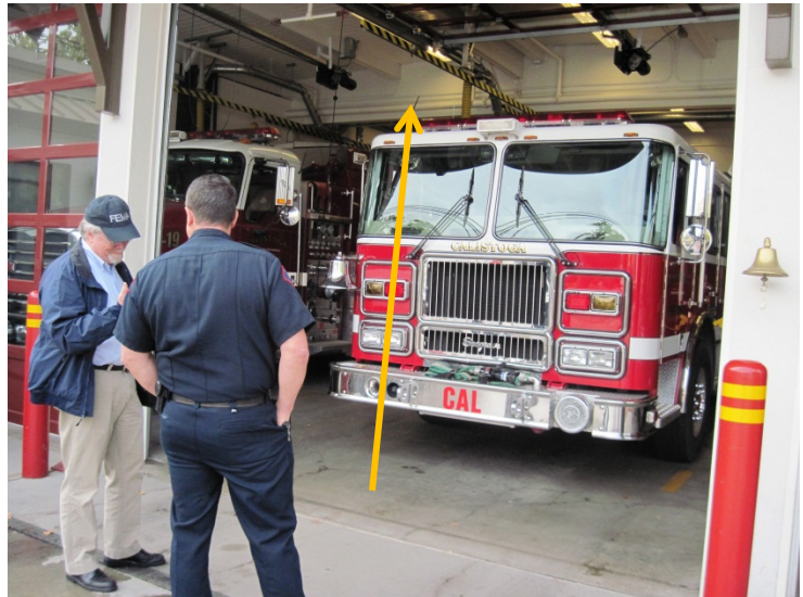
Steve Campbell, Fire Chief calls Mike Mahoney, FEMA Geophysicist attention to the new collector beam installed to collect diaphragm forces and transfer them to new shear wall. (Photo: Bonnie Hanchett)
