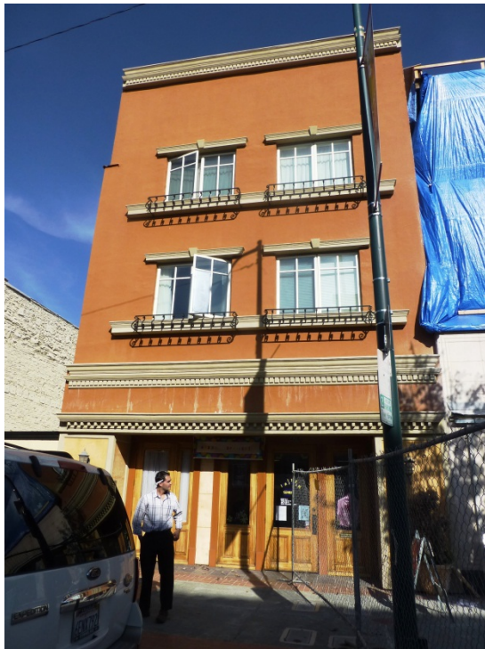
The Casa de Vinci building which was refurbished and seismically retrofitted in 2004 had minimal damage to interior walls. (Photo: Emile Wong)
