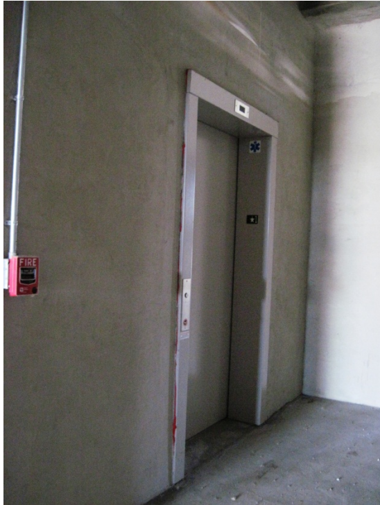
A concrete elevator shaft was installed to serve as a structural pillar (Photo: Bonnie Hanchett)
