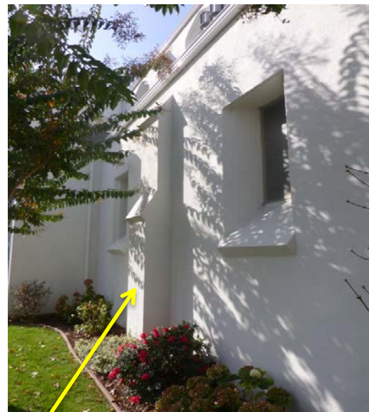
The seismic retrofit included buttresses, like the one pictured above, with Shotcrete and steel reinforcing bars. (Photo: Emile Wong)
