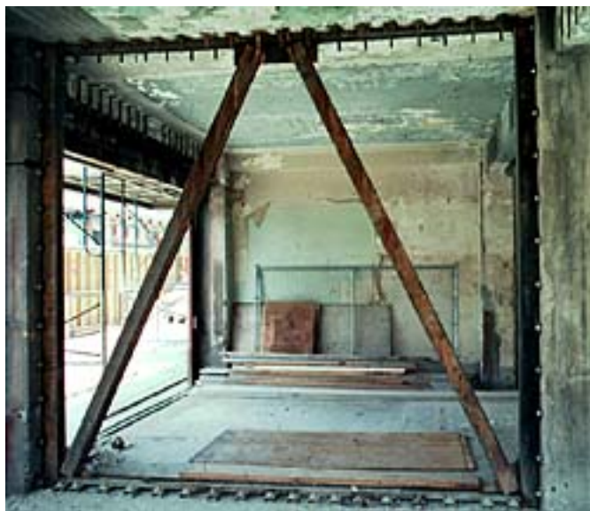
Shown here is an interior diagonal frame which will dampen and transfer seismic loads in a designed path from foundation to roof. (Photo: David Look, American Institute of Architects and published by the National Park Service)
