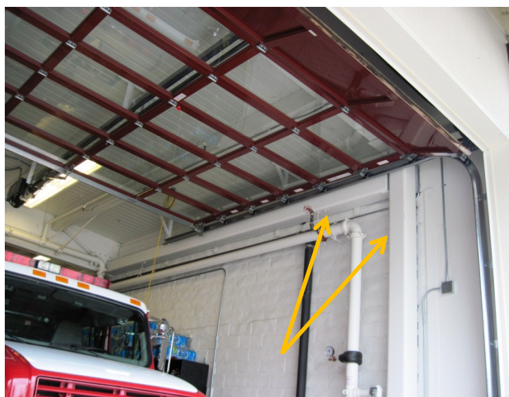
Structural steel members were placed vertically and horizontally on the inside of the masonry walls (Photo: Bonnie Hanchett)
