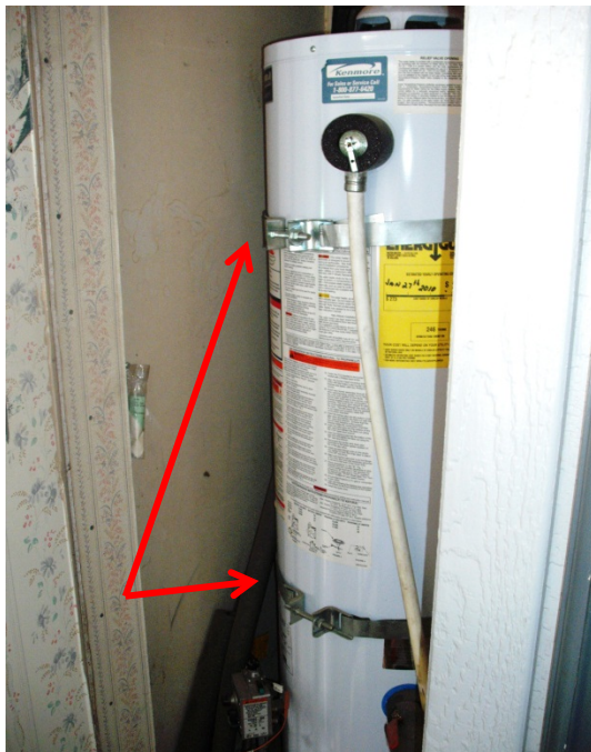
Water heater was braced by strapping it securely to wall. (Photo: Madeline McClure)
