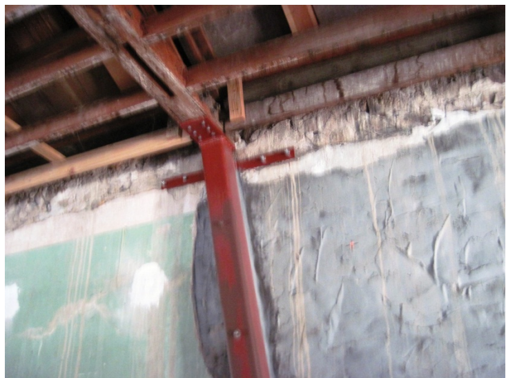
Steel bracing was installed and wall dowels were secured to interior stone walls. (Photo: Bonnie Hanchett)
