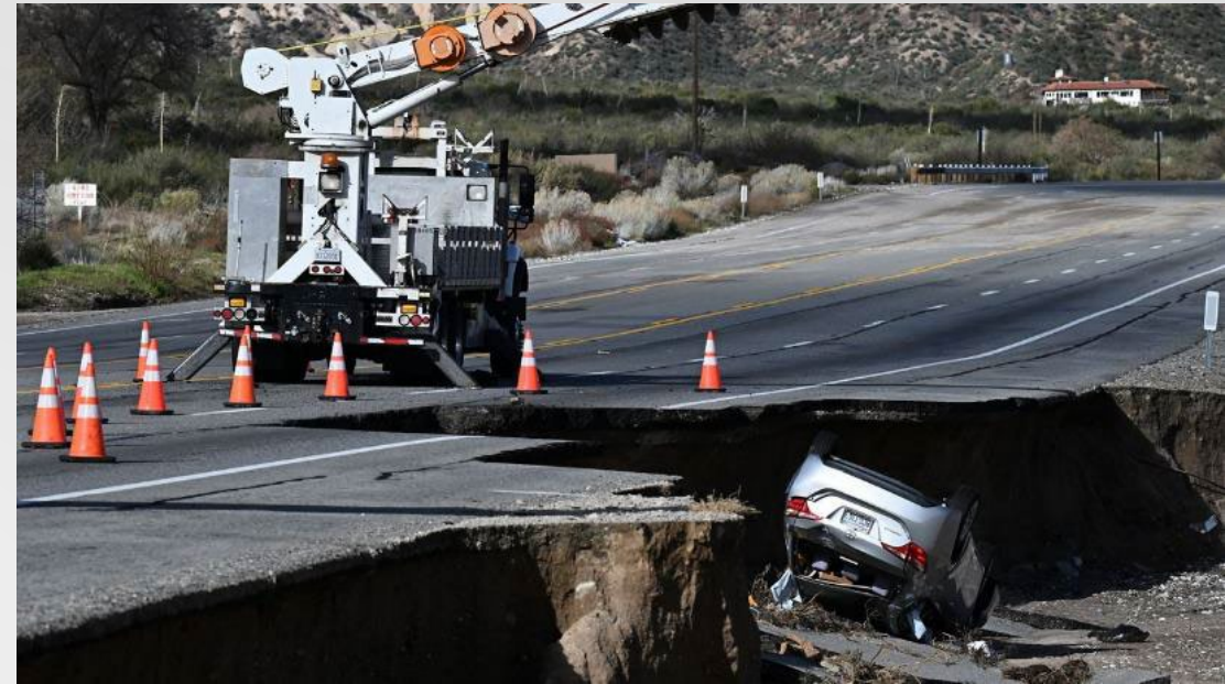
Image: Flood damage on CA-138 south of Phelan, CA, Dec. 2026.
