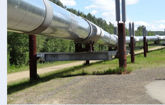
Fuel and Pipeline Damage
