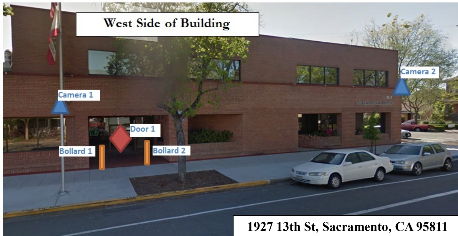
Figure 2. Example of ground-level photograph showing proposed attachment of new equipment
