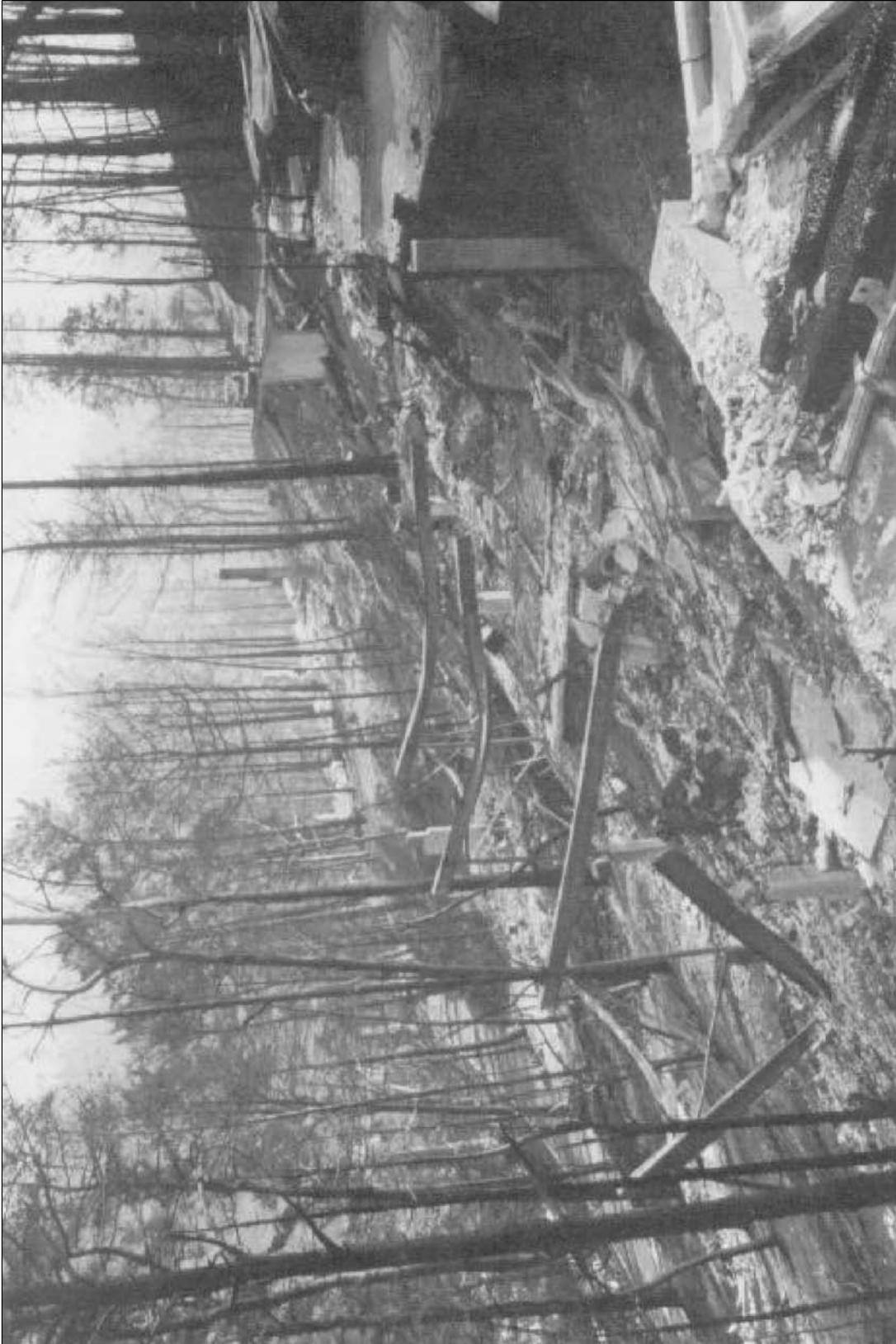
Buckled steel beams mark the location of a destroyed home on Buckingham Boulevard.
