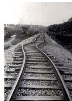
Earthquakes can damage rail tracks, as shown in this 1935 image from the earthquake in Taichu-Shichiku, Japan. Metrolink uses ShakeAlert Messages to automatically slow or stop trains before reaching damaged tracks. Image is courtesy of Wikimedia Commons .
