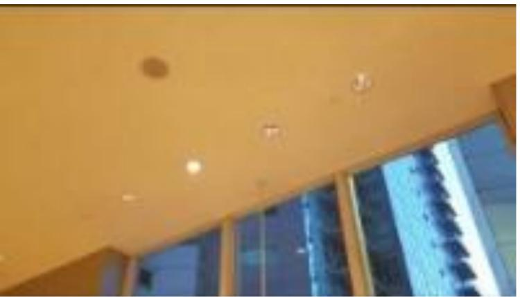
Video of Earthquake Warning Test Residential Condo High Rise (https://www.youtube.com/watch?v=hMOhhaHrKwc) demonstrates a test of an alarm system for an Earthquake in a building. An overhead speaker announces "Earthquake" accompanied by sirens.
