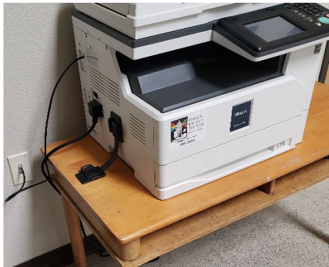
Seismic restraint strap with adhesive fastener used on low bookcase and desktop printer (photo from Humboldt County Office of Education).
