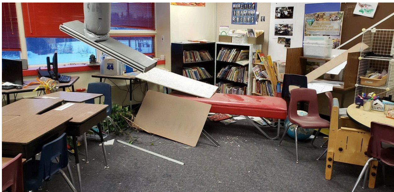
2018 Anchorage Earthquake damage to Matanuska-Susitna Borough School District, Alaska (from Earthquake Engineering Research Institute).
