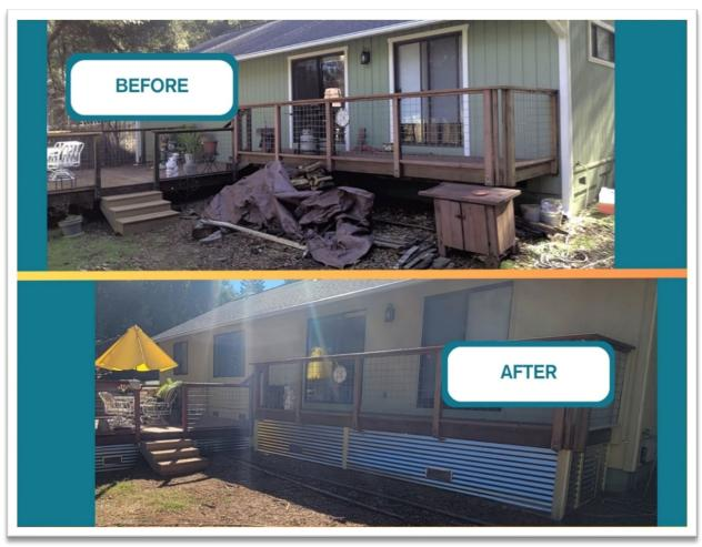
The image above shows a deck that has undergone home hardening retrofits. The space around the deck was cleared of miscellaneous flammable materials and the underside of the deck was fully enclosed. Enclosing the deck prevents flammable materials from accumulating below the deck and prevents flames and embers from igniting the deck from below.
