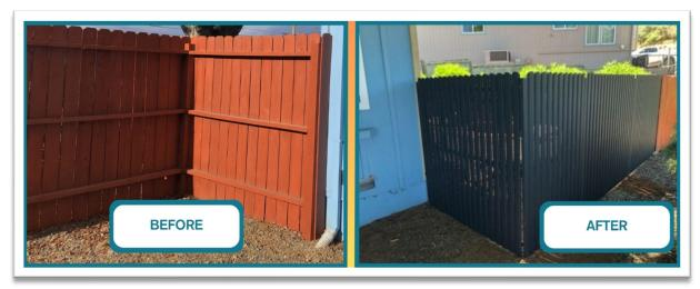
The image above shows an attached fence that has undergone home hardening retrofits. The combustible fencing material was replaced with ignition resistant material within 5 feet of the structure. This prevents fire from spreading along the fence and igniting the wall or eaves of the structure.
