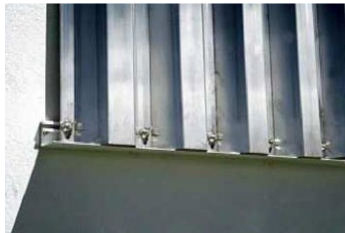
Figure 15. This metal shutter has top and bottom tracks that are permanently anchored to the wall (FEMA 577).
