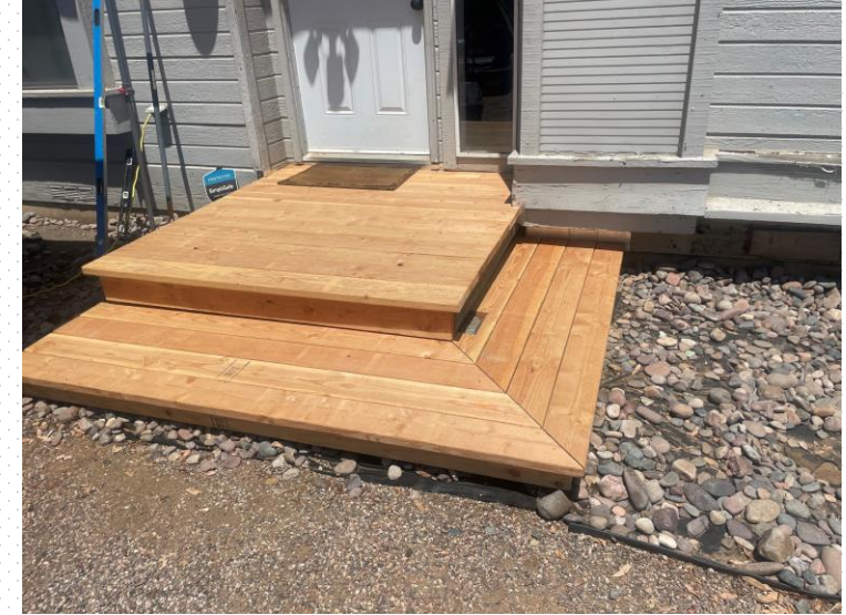
New Deck and Porch built with Fire Treated Lumber
