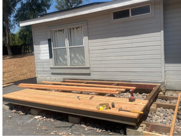
New Deck and Porch built with Fire Treated Lumber
