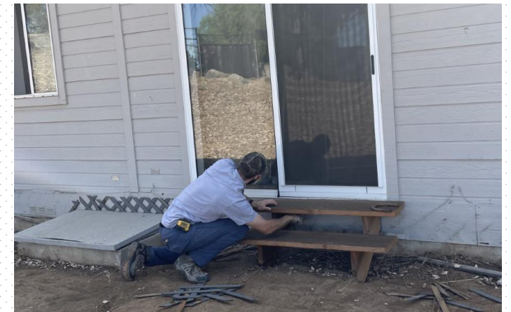
Removing the Combustible Skirting
