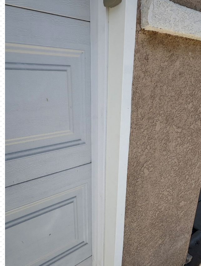
After: Garage door trim replaced with fiber cement trim and new gaskets installed.
