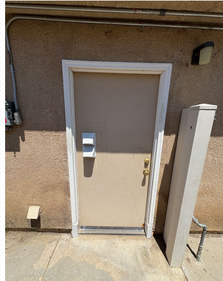
After: Metal door retrofitted with two metal Dryer vents.
