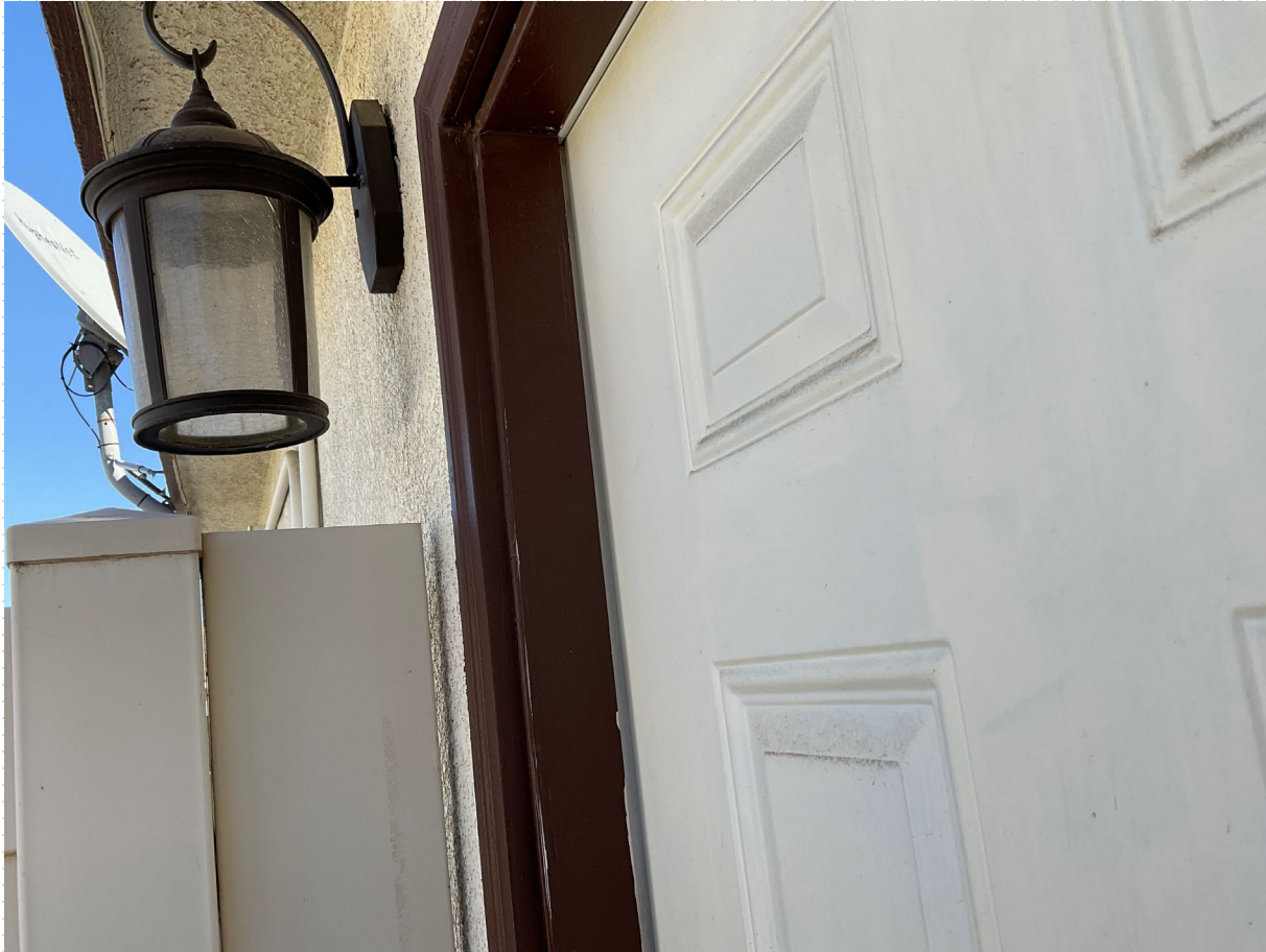
Before: Garage door trim made of combustible material
