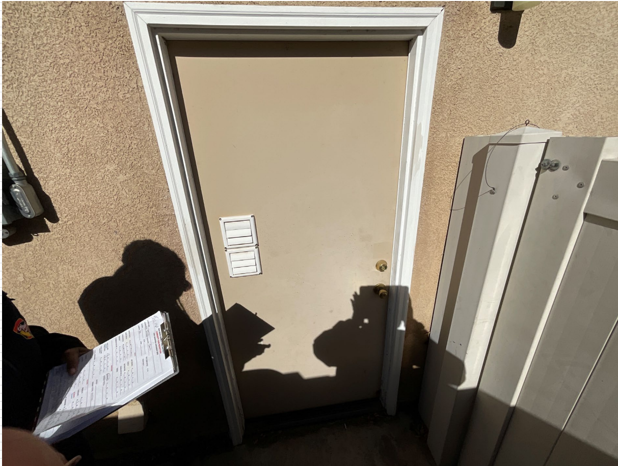
Before: Metal door has two plastic vents:
