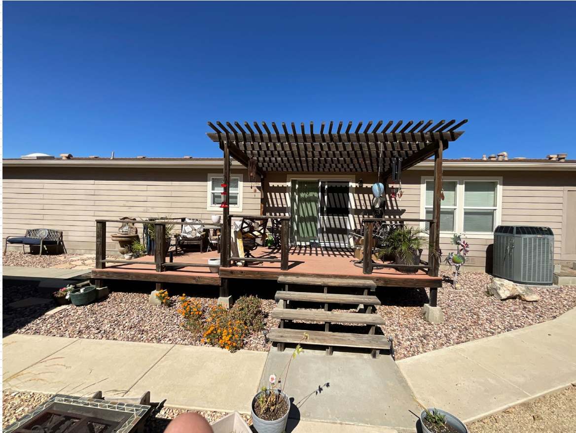
Before Photo of combustible deck boards and pergola
