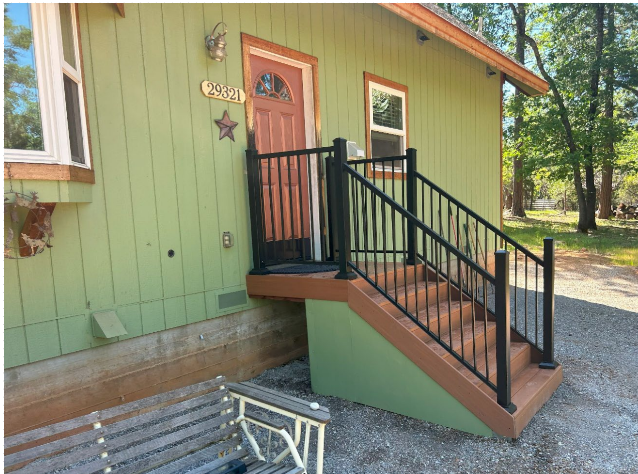
New deck with all non-combustible material
