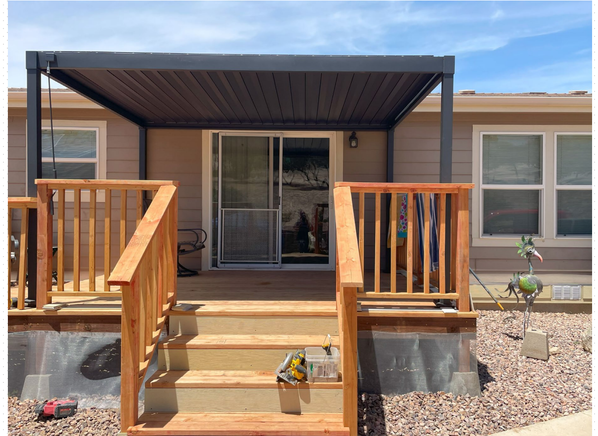
After with non-combustible Fire-X rated treated lumber, fiber cement to close off steps and metal Pergola.
