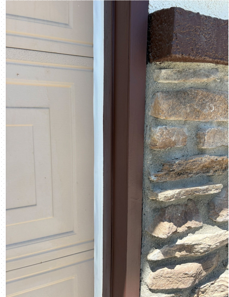
After: Garage door trim replaced with fiber cement trim and new gaskets installed.
