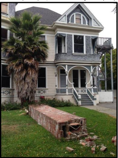
2014 South Napa Earthquake, Non-Structural Damage: Chimney Collapse
