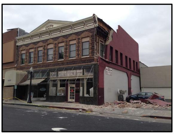
2014 South Napa Earthquake, Unreinforced Masonry Wall Collapse
