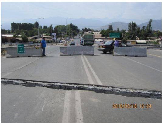
Displacement and Closure of Highway Overpass Following Chile Earthquake
